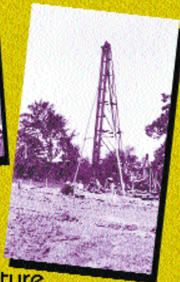
Above: This crane had a single lifting cable, so leads had to be held in place by guy wires. Right: An early Purdy Construction project. The hammer appears to be a Vulcan 50-C.
