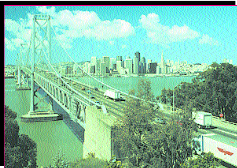
San Francisco's Bay Bridge
