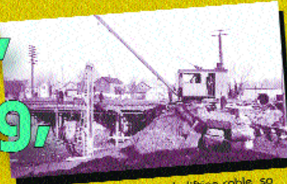
Above: This crane had a single lifting cable, so leads had to be held in place by guy wires. Right: An early Purdy Construction project. The hammer appears to be a Vulcan 50-C.
