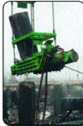
16" PCPC & 2-Part Cradle removing a pile cutoff
