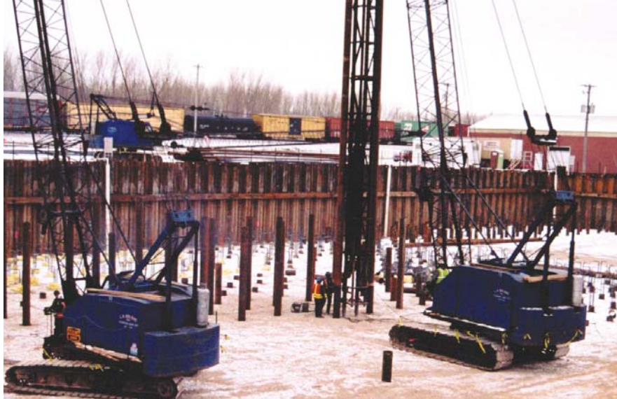
L.H. Bolduc Co. mobilized multiple rigs to increase production.
