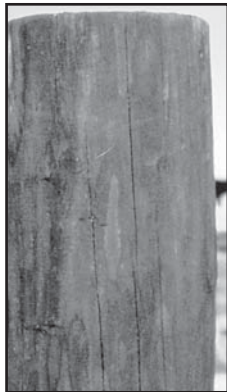
BMP TREATED PILING
