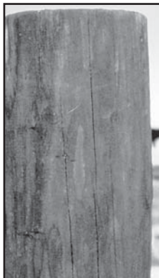
BMP TREATED PILING
