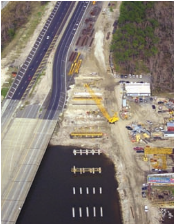
Image of work on I-10 near Lake Pontchartrain.
