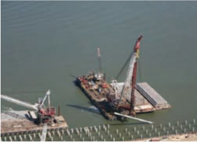
The Weeks 526 pending a 54" diameter cylinder pile.
