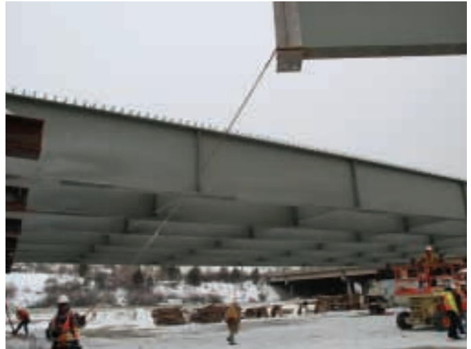
Setting girders for one of the bridges in the bridge farm.
