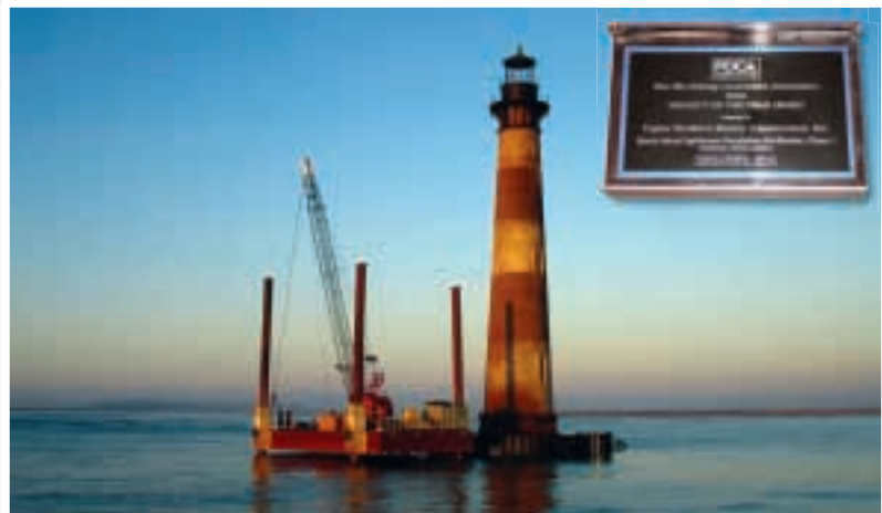
The Pile Driving Contractors Association 2009 Project of the Year - Greater than $2 Million.
