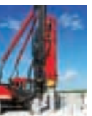
On the Cover: Junttan rig driving concrete piles
