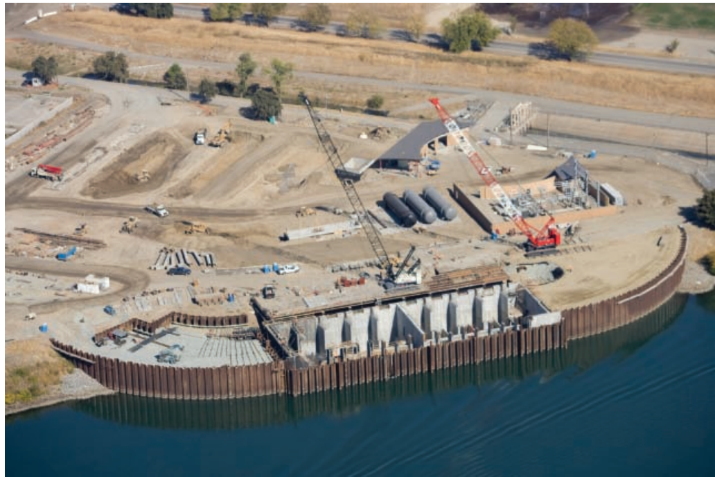
Figure 4: The combi-walls support the construction of the treatment facilities concrete structure
