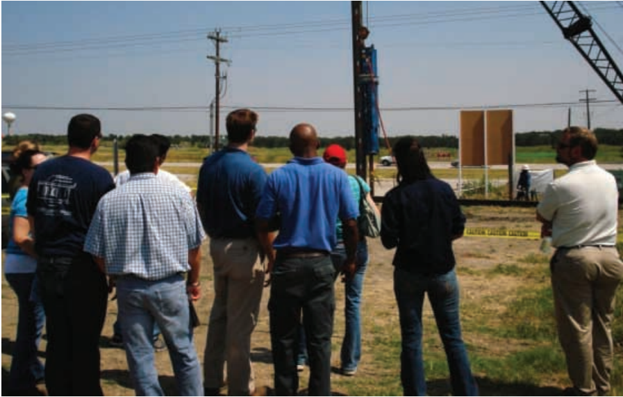
The Pile Master 36-3000 driving a 6-5/8 inch, 25 ft long pipe pile in Manor, TX
