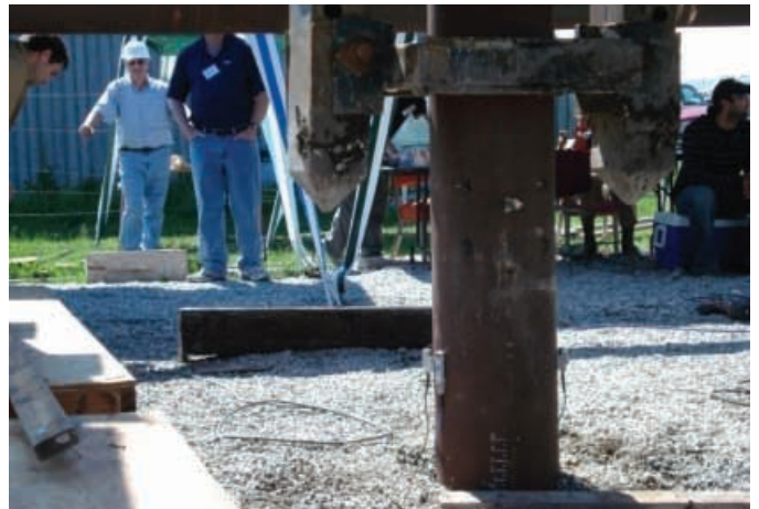
Pile Driving and testing demonstration in Austin, TX
