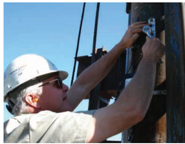
PDPI instructor Pat Hannigan installs wireless gages
