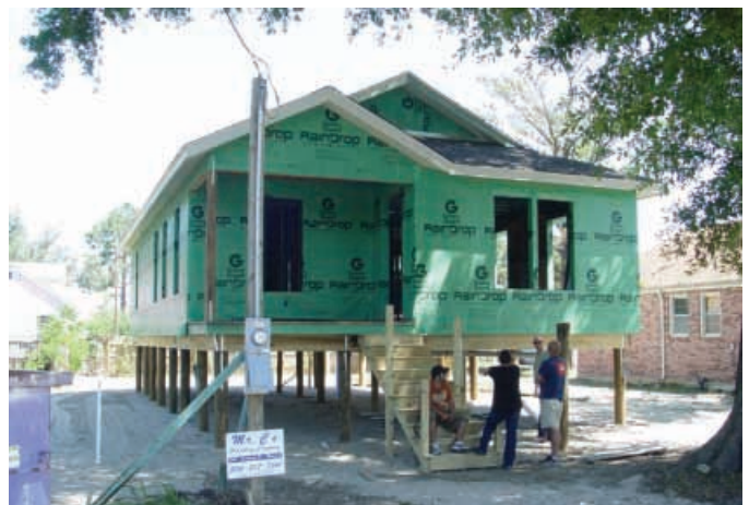
The home at 840 Pontalba Street in New Orleans defines the strength and beauty possible when building with timber pilings.
