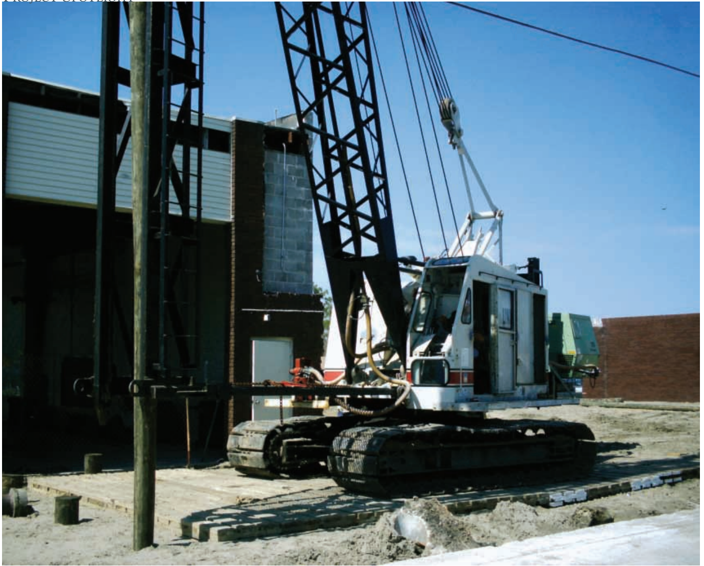
Dmitri often drives residential pilings with a C-350 Bantam.
