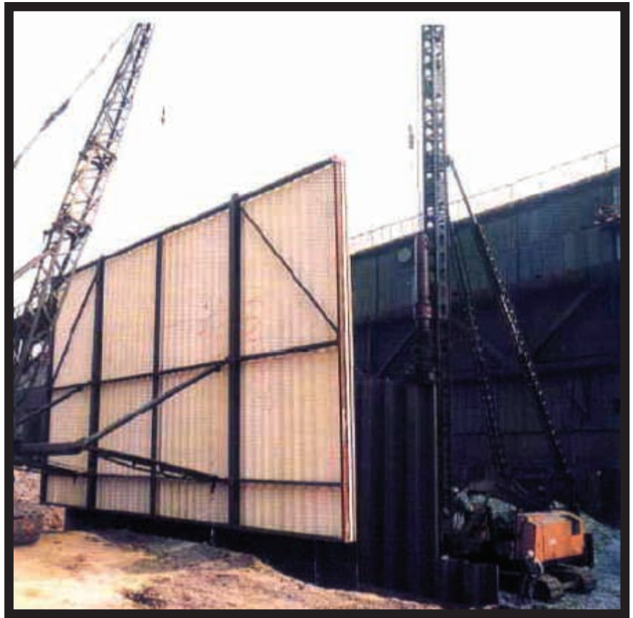
Figure 2. Screening can reduce the amount of noise from pile driving
