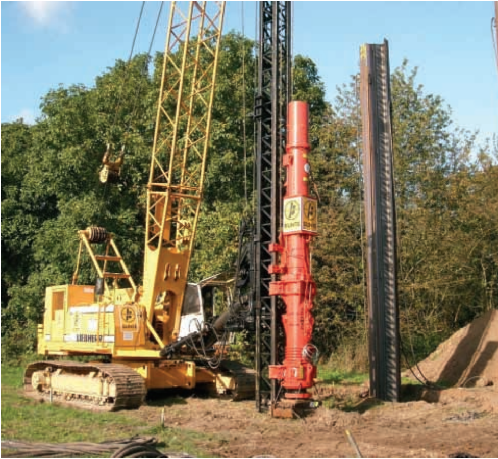
Figure 3. Precision alignment for closure of cofferdams
