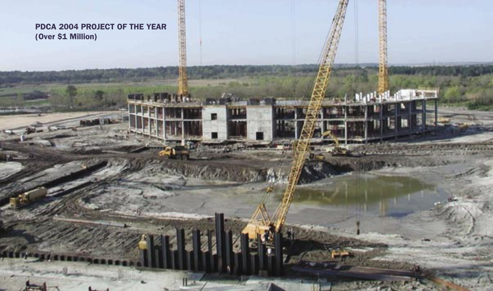
Installation of steel sheet pile to construct casino vessel basin.
