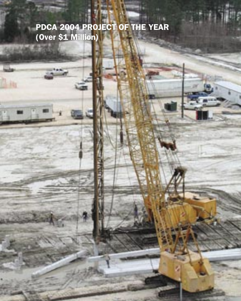
Installation of prestressed concrete bearing pile.
