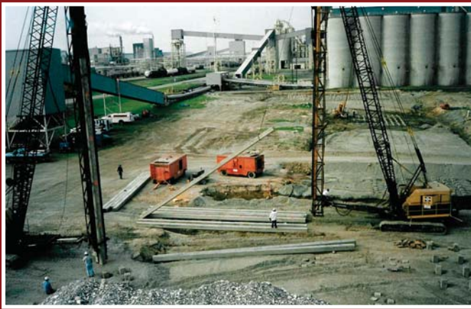
A precast, prestressed pile is hoisted into position for driving at the site.
