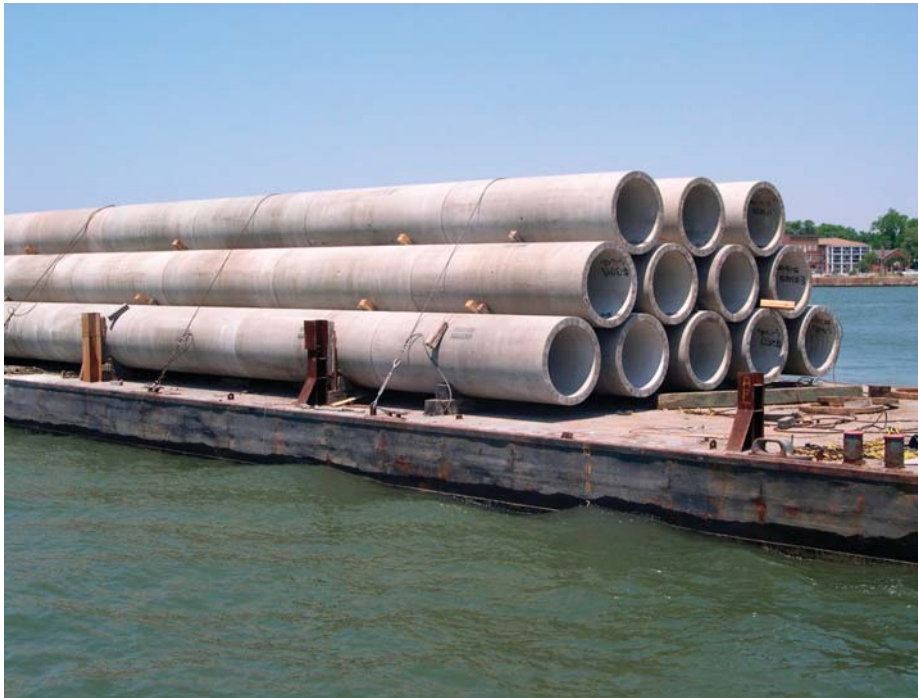
In some cases with bridge projects, transporting the precast piles by barge creates an efficient approach.
