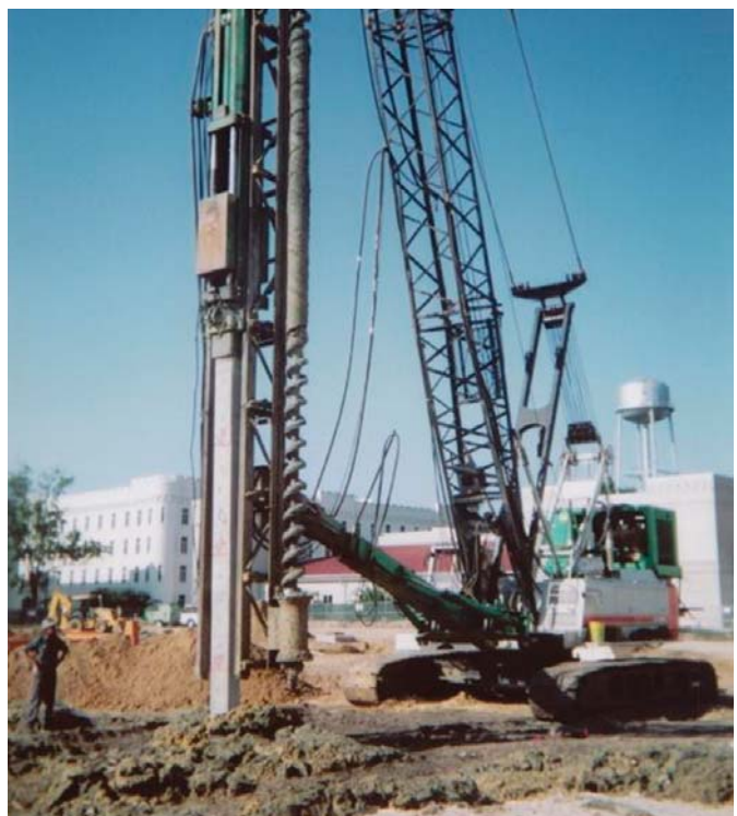
This 12-inch, 85-foot-long precast, prestressed pile is being driven with a hydraulic hammer that includes an auger on the side so the pile can be dropped into a 55-foot-deep hole prior to driving it.
