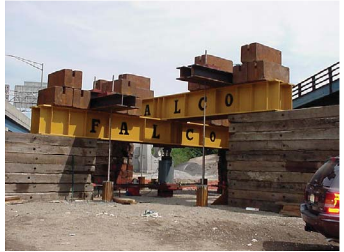
Static Pile Load Test
