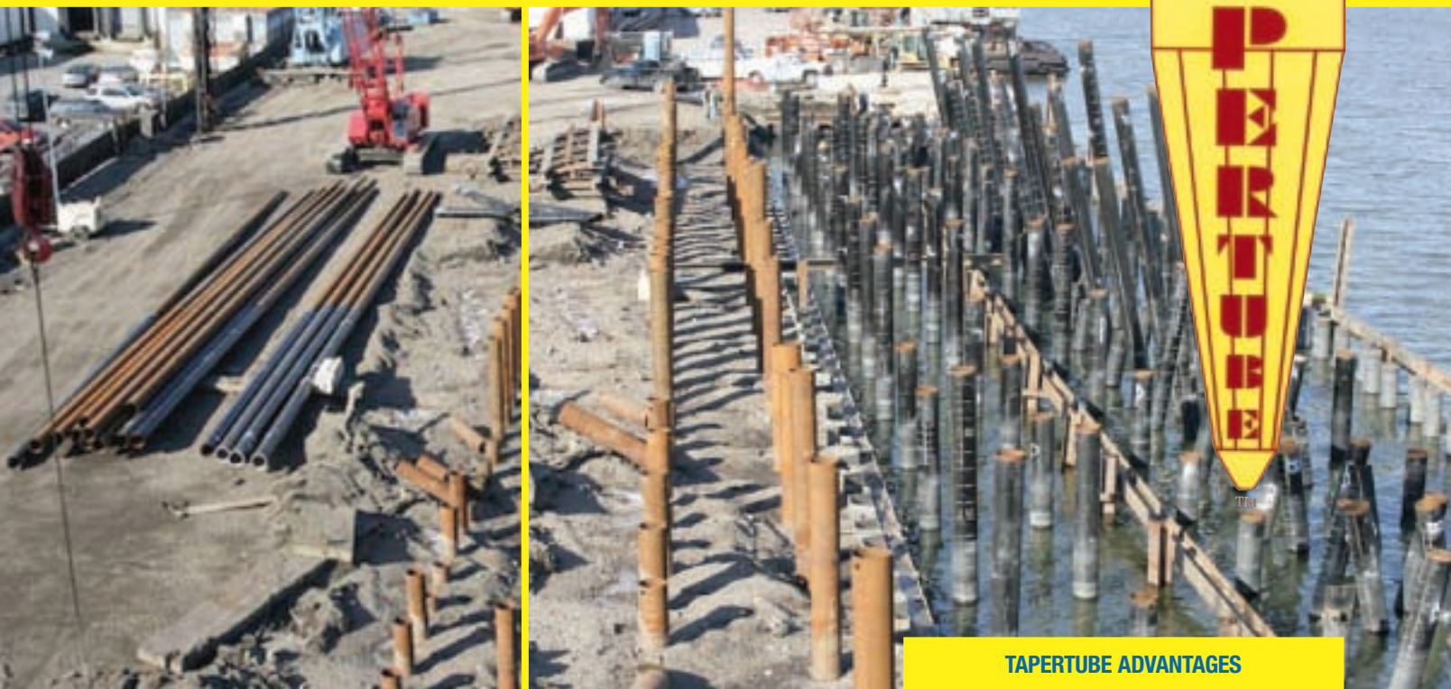
Port of Wilmington Job – Reconstruction of Berth #4 – Kuhn Construction
