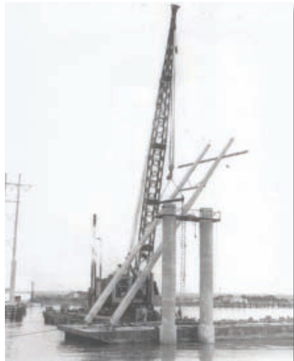
1965 - Beaufort, MC Power Structures. PMCC installed 66-inch prestressed caissons, inserted 54-inch in them, then 100-foot long poles above them.
