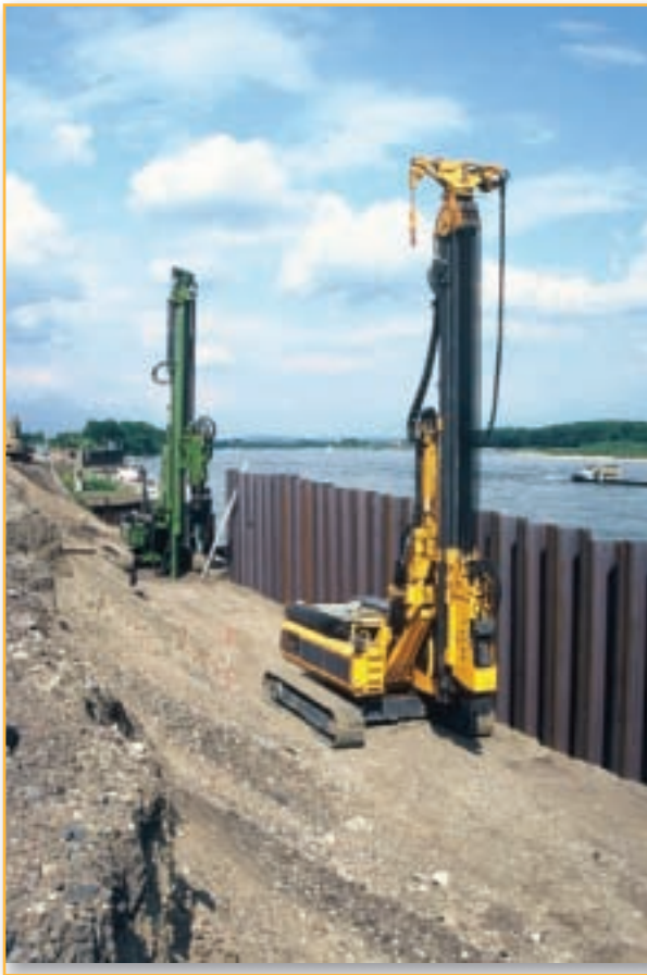
Figure 1: Installing steel sheet piling depends on proper placement procedures for the particular application and soil type involved.
