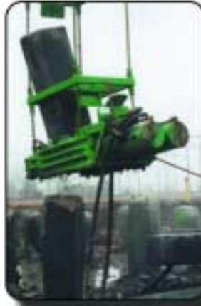
16" PCPC & 2-Part Cradle removing a pile cutoff
