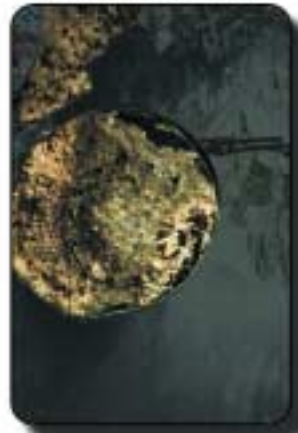
The 36" PCPC cutting a 43" caisson below 15' of water at mudline. The caisson had a 1/2" steel wall & 13 - 1 1/2" rebars.
