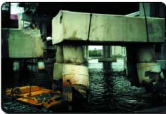
A 34" pilecap with 14" steel H beams cut with a 30" PCPC.
