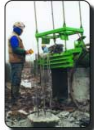
An operator with remote exposing steel strands
