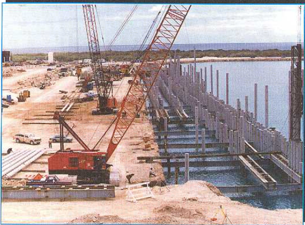
Hawaiian Dredging does its work at Barbers Point Harbor in Oahu, Hawaii.
