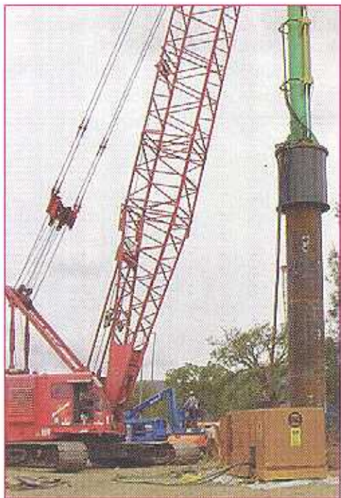
A Manitowoc 4000 crane and Lucas Marine's LMC 50 hydraulic impact hammer driving a 60-inch pile at Putah Creek.
