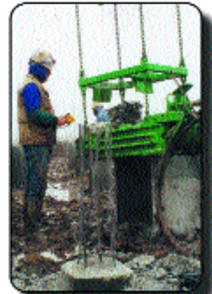
An operator with remote exposing steel strands
