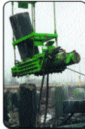
16" PCPC & 2-Part Cradle removing a pile cutoff
