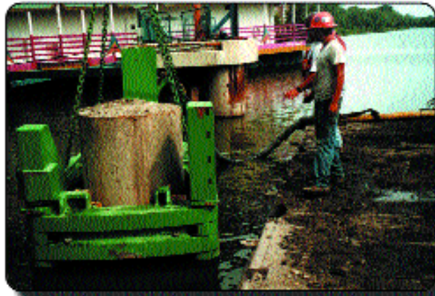
The 36" PCPC cutting a 43" caisson below 15' of water at mudline. The caisson had a 1/2" steel wall & 13 - 1 1/2" rebars.
