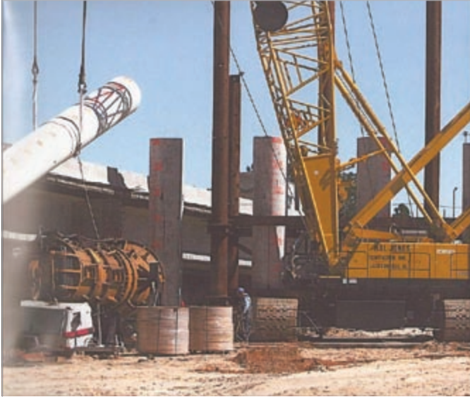
54" concrete cylinder pile being lifted for installation.
