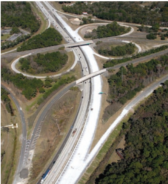
Aerial shots of the Trout River Bridge project.
