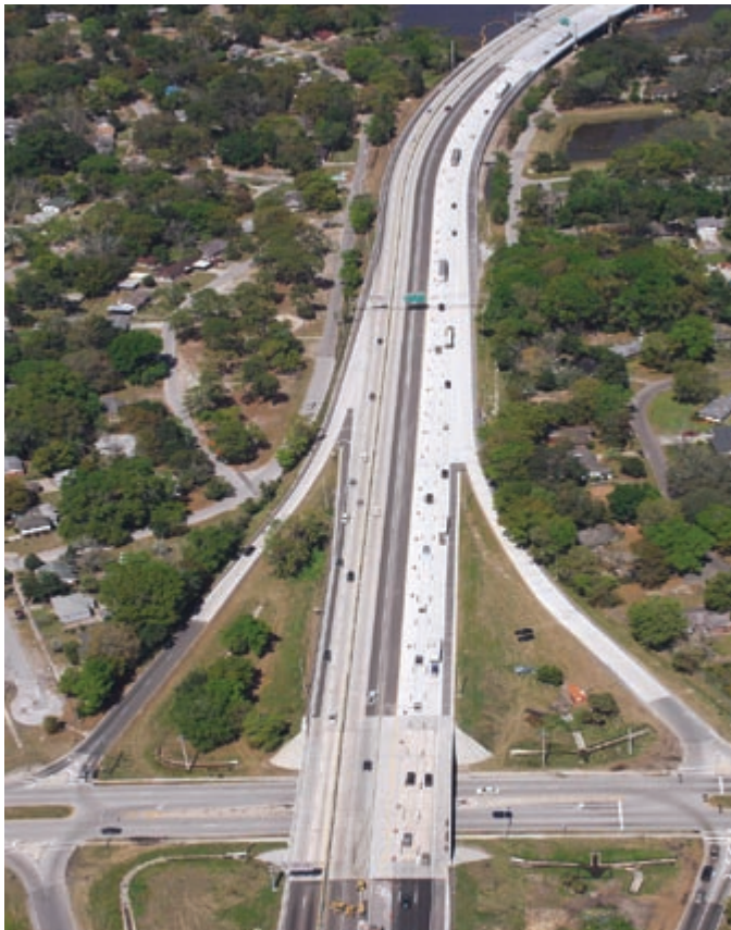
An aerial shot of the Trout River Bridge project.
