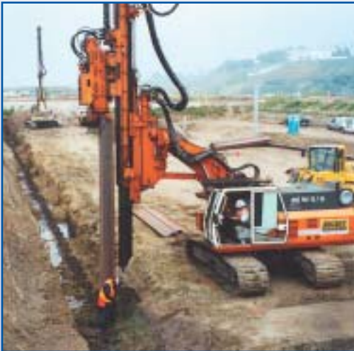
50 pair of sheet pile in 1 day
