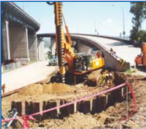
Pre-drilling over 1500FT/day; swaps to hammer in 5 minutes
