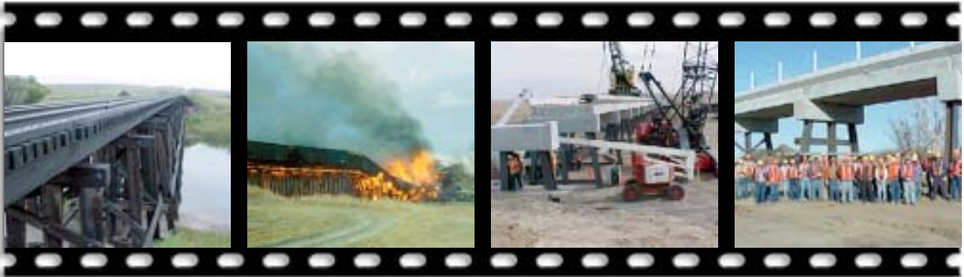
The Sharon Springs Bridge before the fire.
