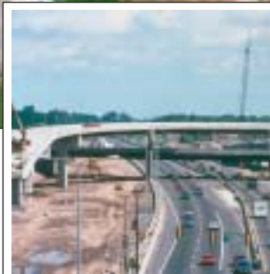
Traffic maintained through all construction phases.
