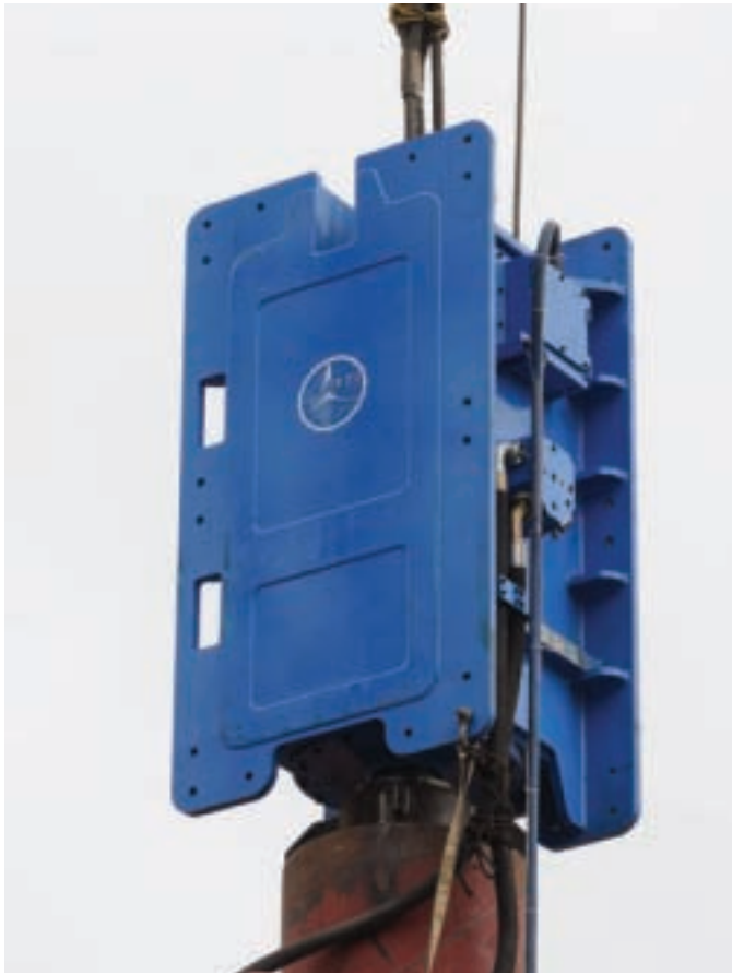
The RD260 Resonant Driver driving a 914 mm dia pipe pile.
