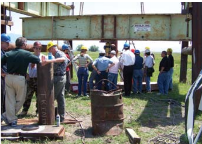
Professors inspect a load test reaction stand
