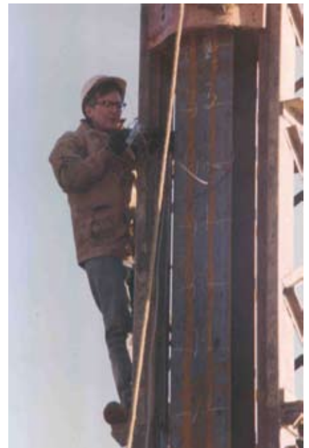
Gage installation in the 1970s
