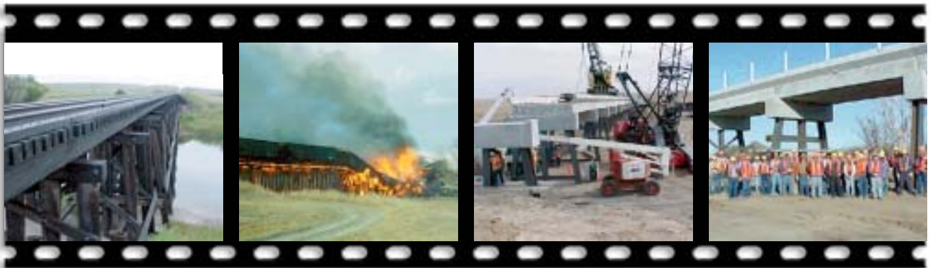
The Sharon Springs Bridge before the fire.
