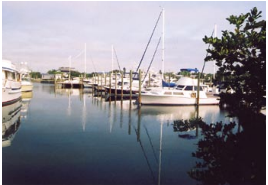
Timber piling is the mainstay for small boat marinas.
