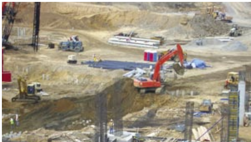
Clark Foundations works on the Washington Nationals ballpark in Washington, D.C.
