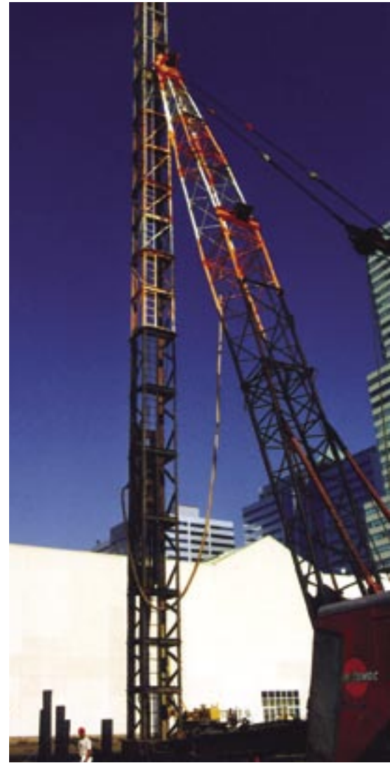
Driving timber piles at a shopping center in New Jersey.
