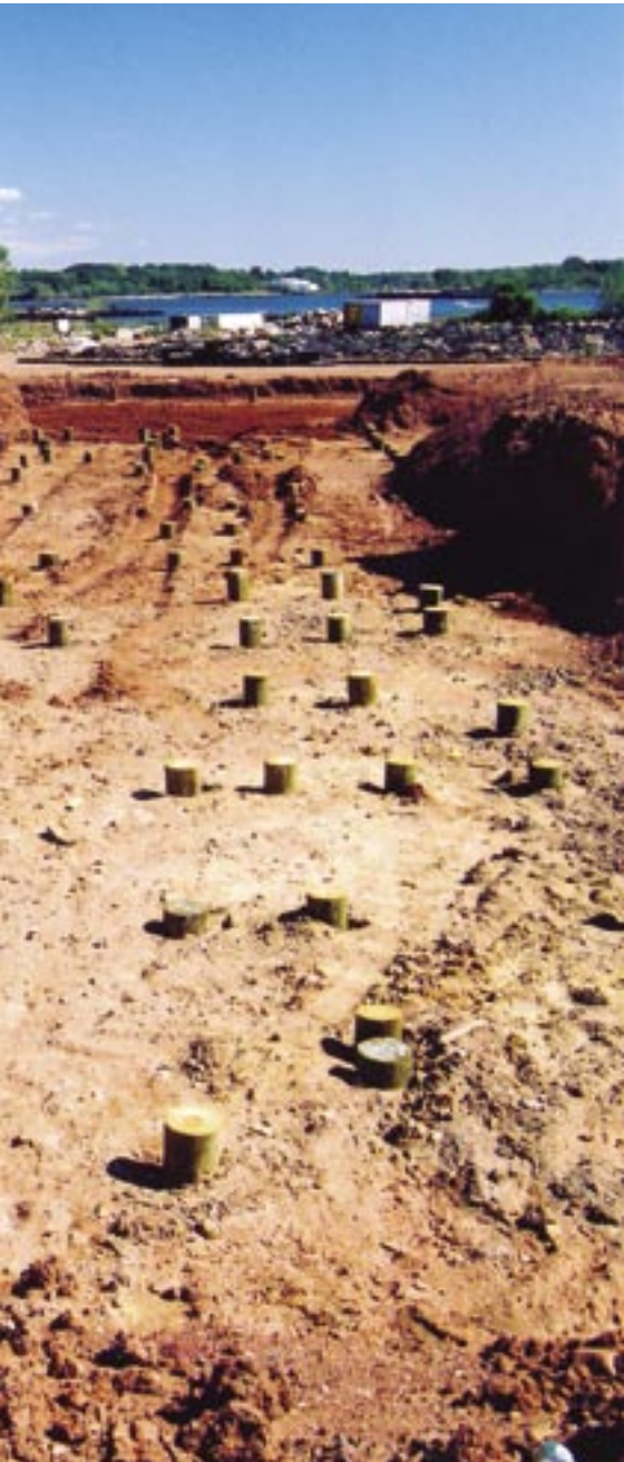
Timber foundation piling system for New Jersey condominiums.
