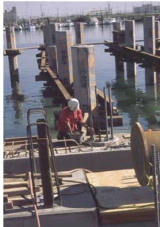
Wharf Construction - Structural fuse can be seen in foreground.
