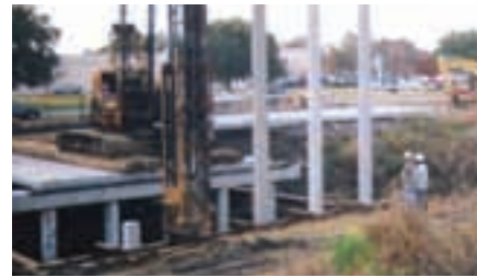
Precast bridge installation at subdivision entrance in Chalmette, La.
