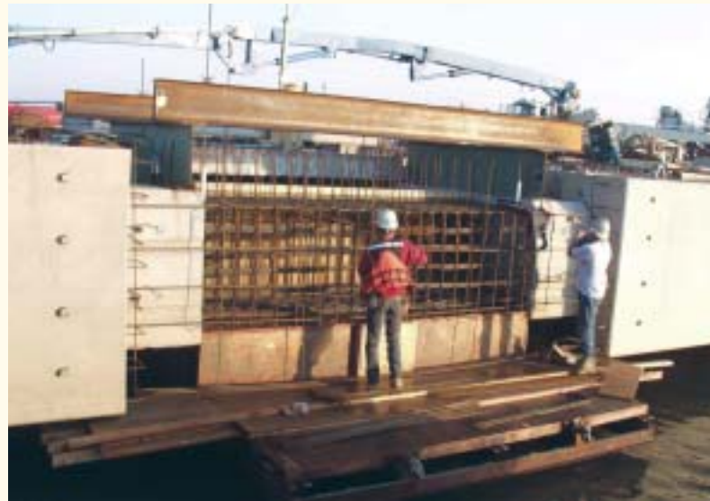
Photo: Kuhn Construction Company
