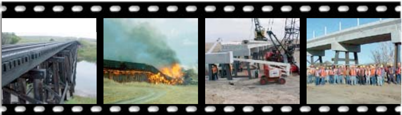
The Sharon Springs Bridge before the fire.
