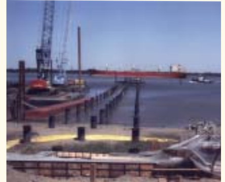
Photo: Kuhn Construction Company
