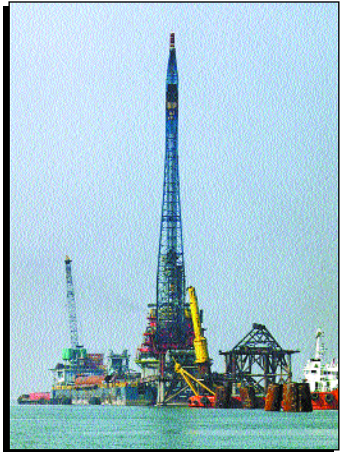
Tubular piles are driven on the Jamuna River in Bangladesh.
