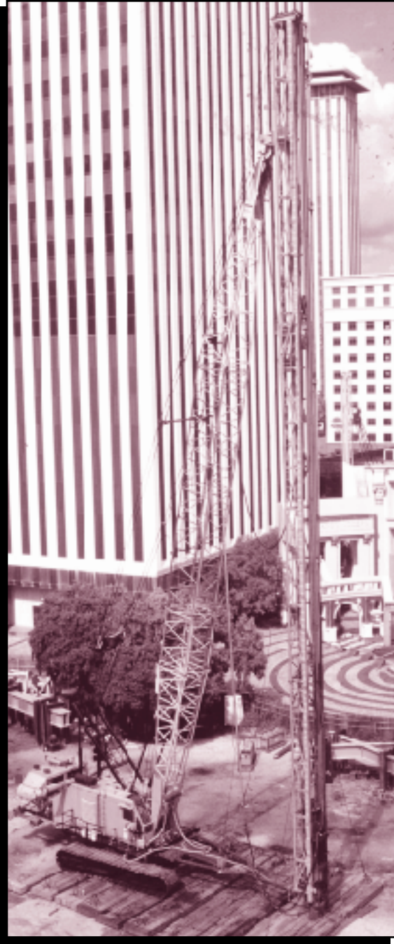
The Westin Hotel in New Orleans was a Boh Bros. project.
