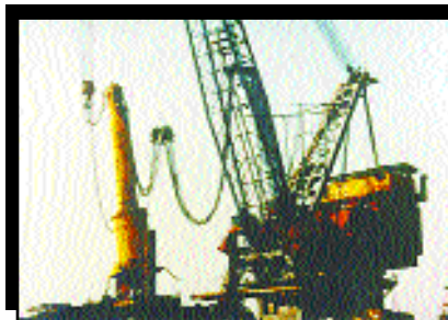
A hydraulic hammer developing 1,230,000 ft. lbs.
