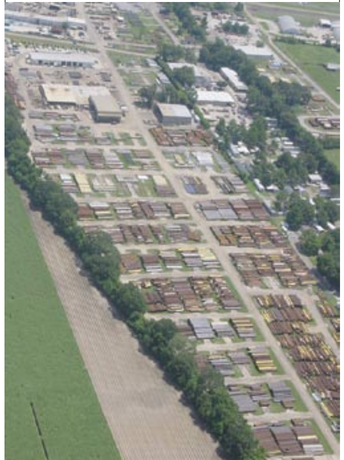
One of three pipeyards located in Lafayette, LA
