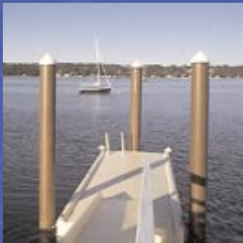
Pearson Pilings Last.
