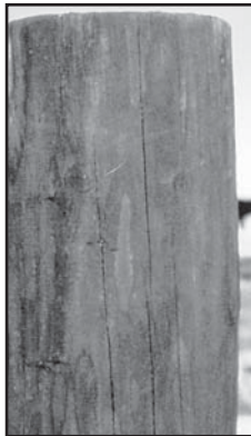
BMP TREATED PILING
