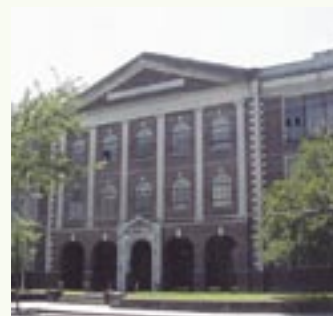
COVER: Project Spotlight: Charleston High School Renovation Project
