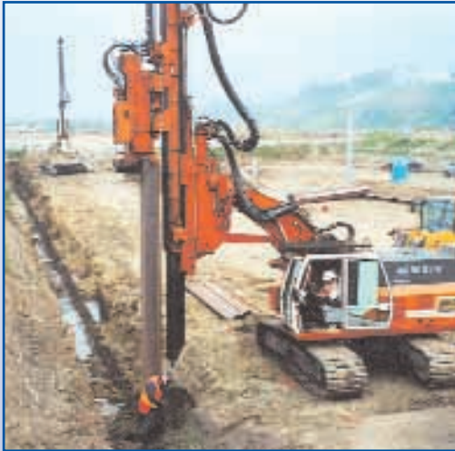
50 pair of sheet pile in 1 day
