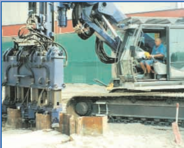
Pre-drilling over 1500FT/day; swaps to hammer in 5 minutes
