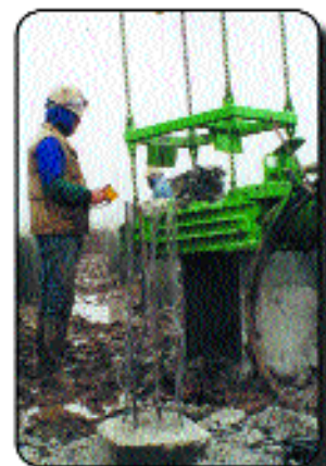
An operator with remote exposing steel strands
