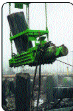
16" PCPC & 2-Part Cradle removing a pile cutoff
