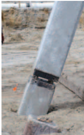
Joining of battered pile splices.
