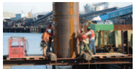
One of the completed new NGC breasting dolphins.
