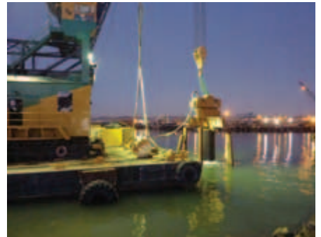
A night shot showing the vibrating of one of the monopiles.
