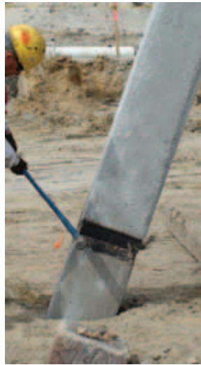
Joining of battered pile splices.
