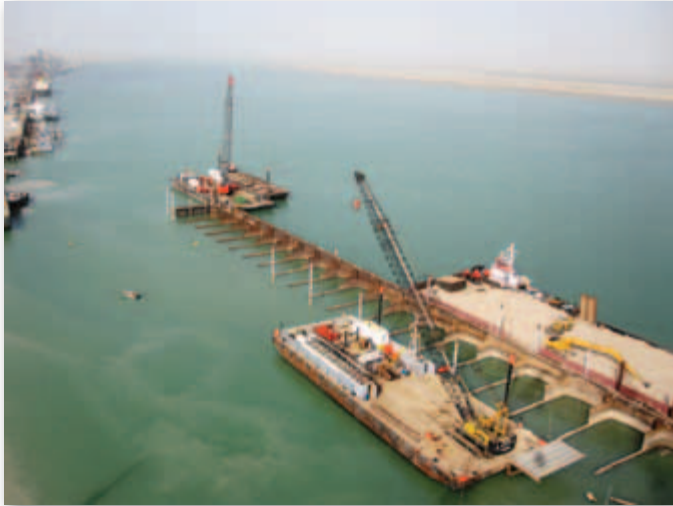
Figure 2: OPEN CELL Seawall under construction.
