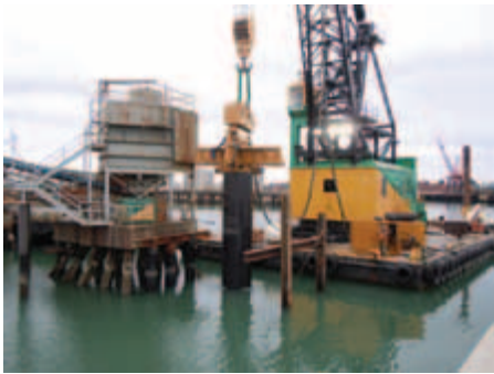
The overall equipment involved in the project; barge, crane and hammer.
