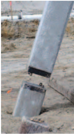
Joining of battered pile splices.
