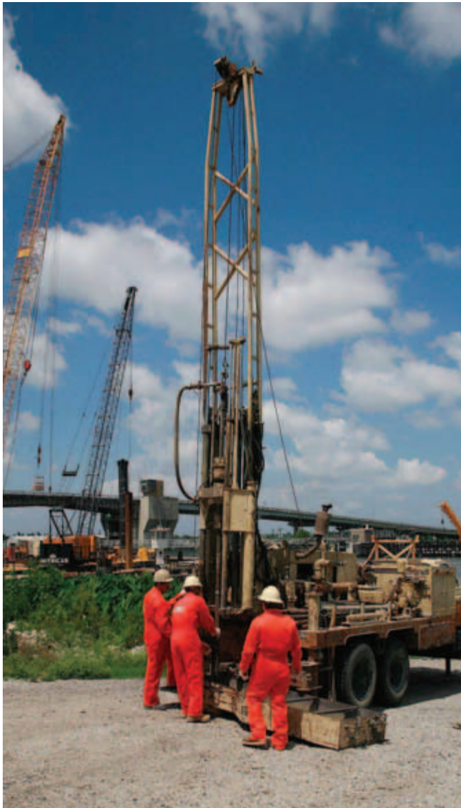
Fugro collecting Data on the New Orleans Storm-Surge Protection Levees.
