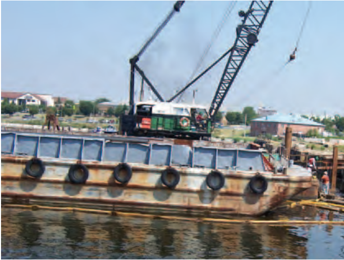
Installing sheet piles at Canton Crossing in Baltimore, Maryland.
