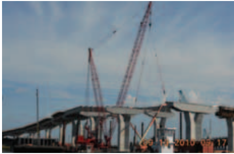
Beam Erection Piles under footings
