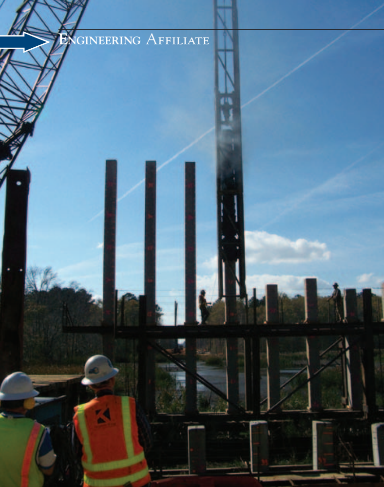
Above: Construction of a new ferry terminal for Bald Head Island in eastern North Carolina. S&ME provided site characterization services, foundation recommendations, dynamic pile testing and construction support.
