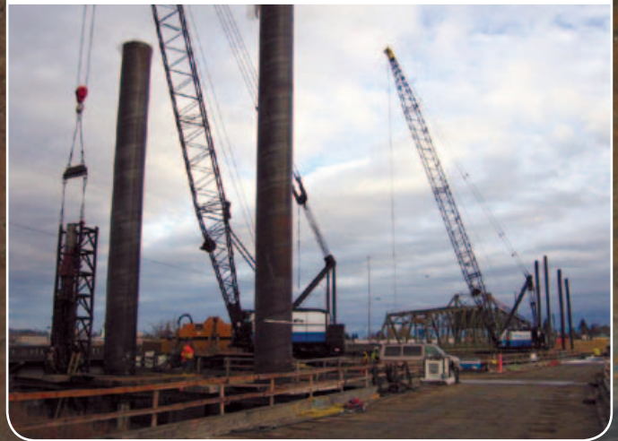
Ebey Slough Bridge Replacement
