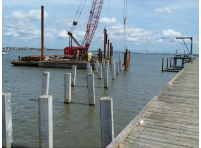
Above: Prestressed concrete piles being driven by PDCA member Cape Romain Contracting for a new dock at the James Island Yacht Club in Charleston, SC. S&ME provided geotechnical engineering services, including dynamic pile testing.
