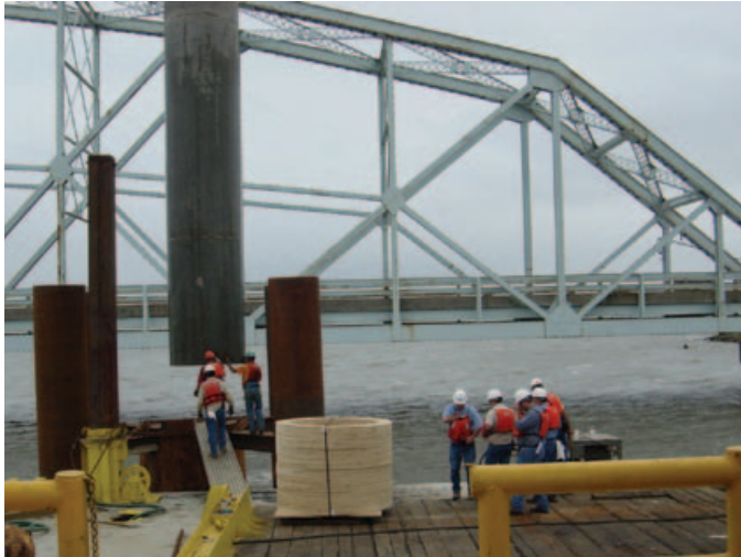
Rigolets Bridge – 66 Inch Test Pile O11
