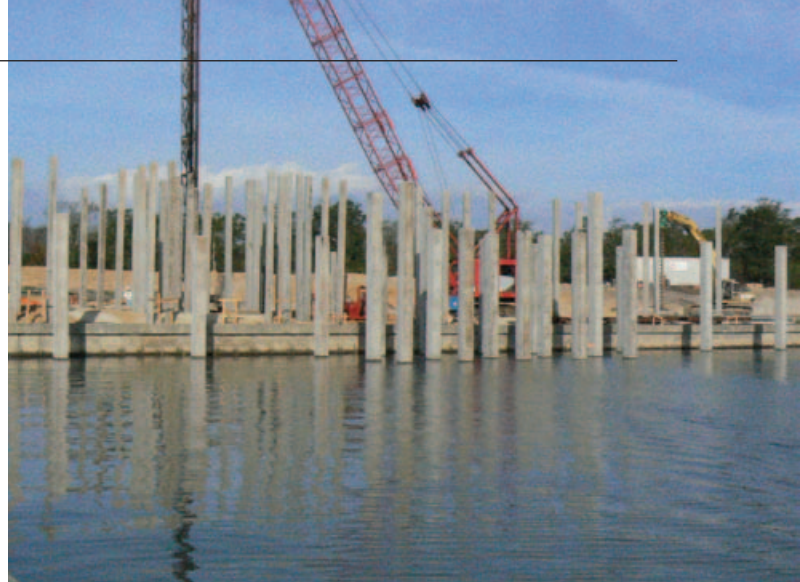
Above: Construction of a new ferry terminal for Bald Head Island in eastern North Carolina. S&ME provided site characterization services, foundation recommendations, dynamic pile testing and construction support.
