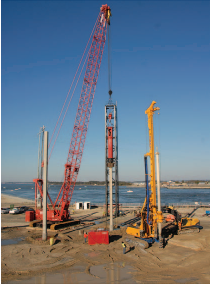
Above: Prestressed concrete piles being driven by PDCA member Cape Romain Contracting for a new dock at the James Island Yacht Club in Charleston, SC. S&ME provided geotechnical engineering services, including dynamic pile testing.
