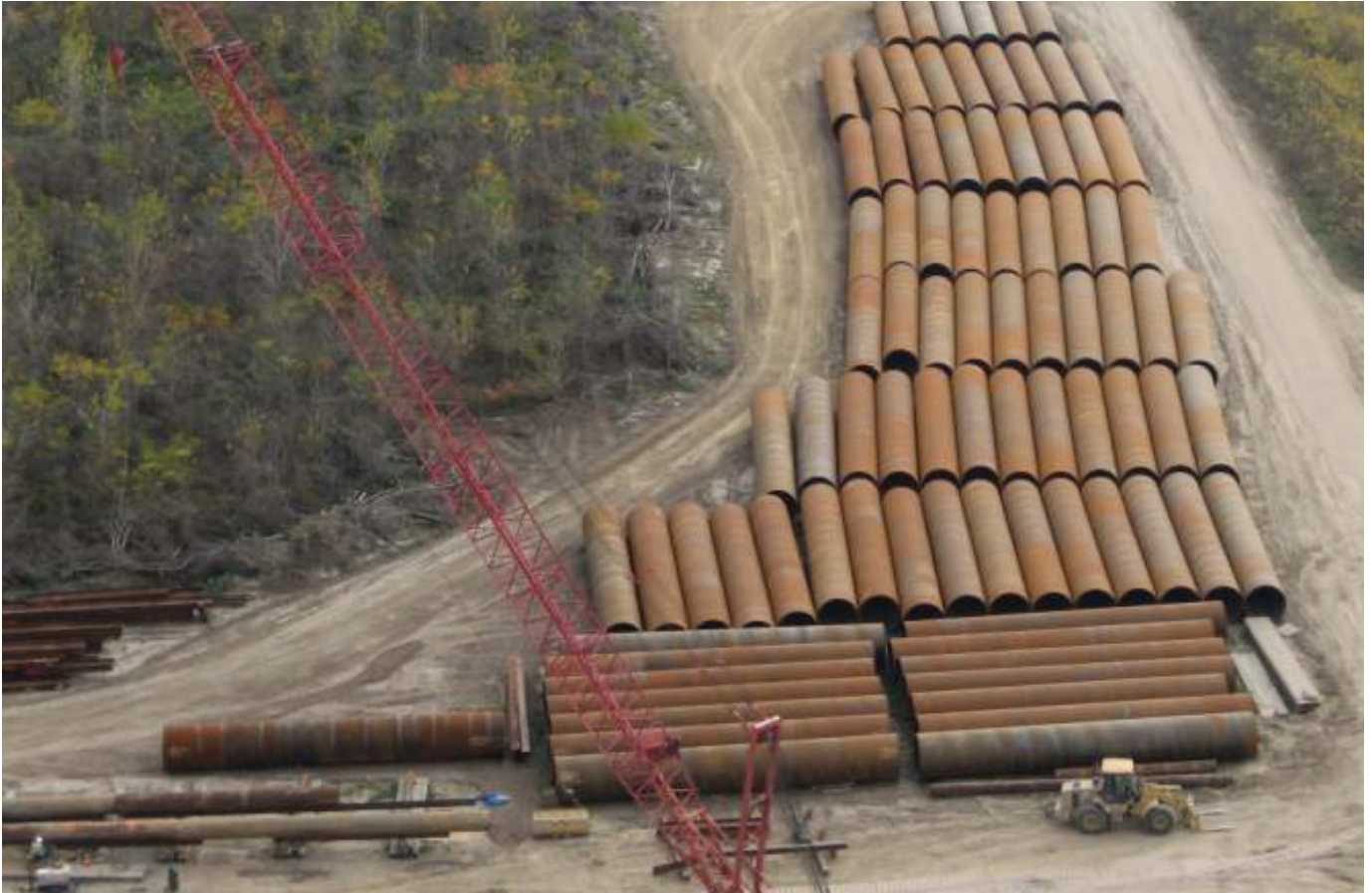
96" diameter pipe is assembled alongside the Mississippi River for the foundation of the John J Audubon Bridge, which, upon completion, will be the longest Cable Stay Bridge in America.
