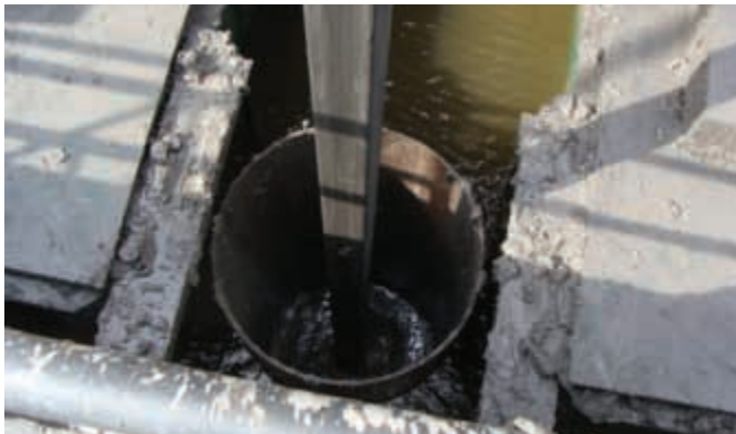
Figure 11. Casing Located in Barge Slot
