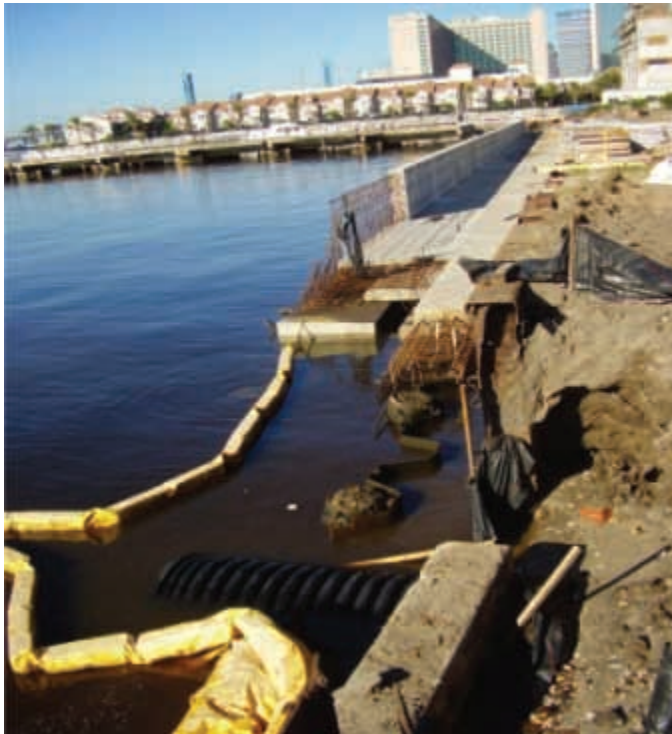
West end portion of the completed shipyards.
