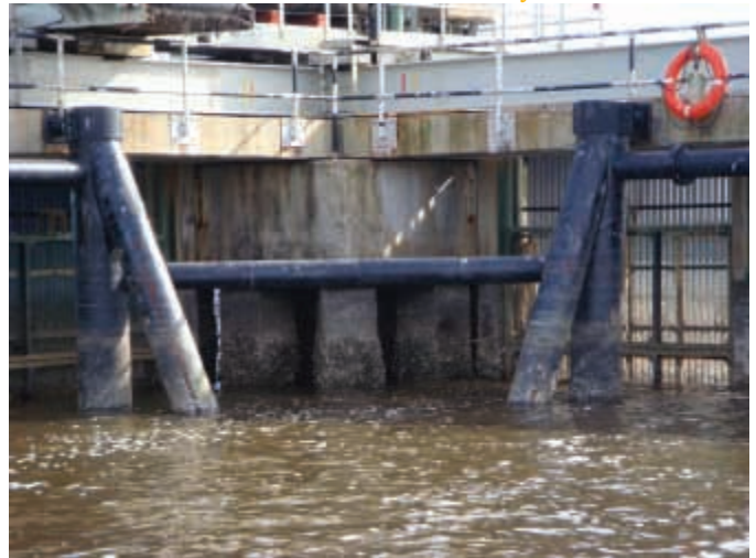
Figure 13. Pile Connections to Structure
