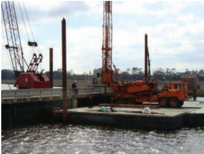
Figure 10. Crane Barge Supporting Drill Rig
