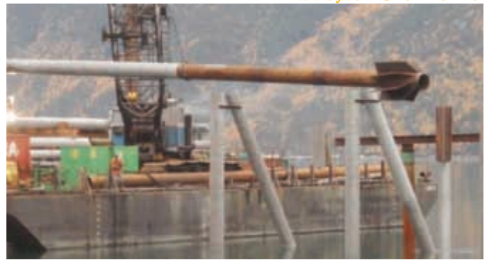
Loading Bearing Pile
