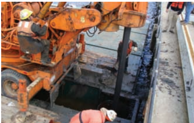
Figure 12. Drill Rig on Shugart Barges with Slot
