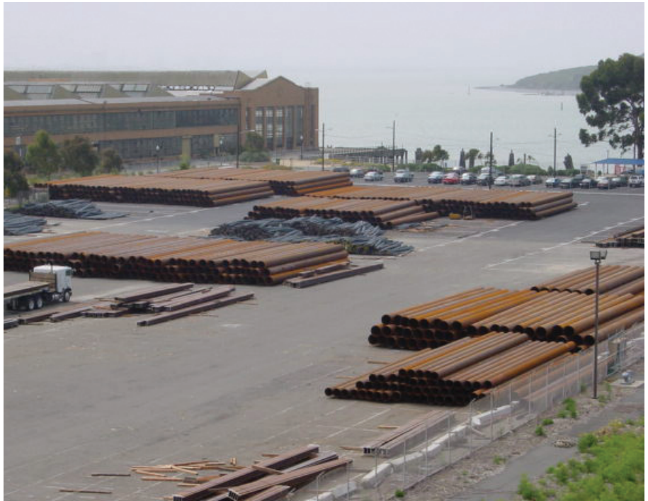
6,000 tons of 30" diameter heavy wall steel pipe assembled on the dock in Richmond, California destined for the foundation of the New Carquinez Bridge.
