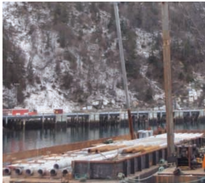
Preparing Barrier Piles to be Driven
