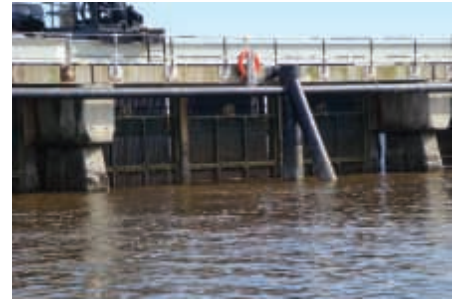
Figure 8. Damaged H-Pile
