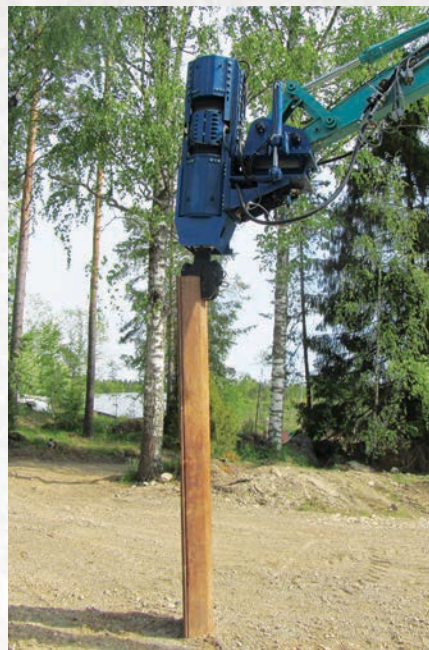
Driving into hard silt or extracting the pile
