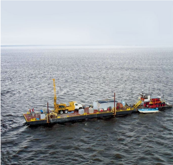
Geotechnical drilling being performed at Choctawhatchee Bay
