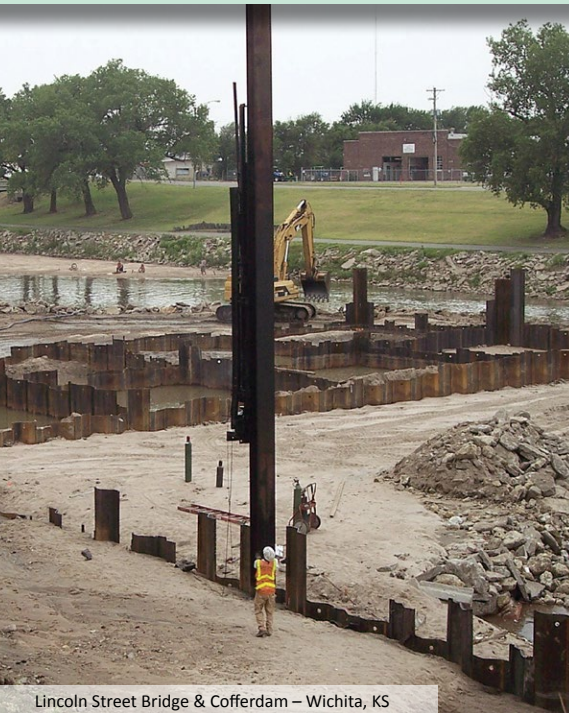
Lincoln Street Bridge & Cofferdam – Wichita, KS
