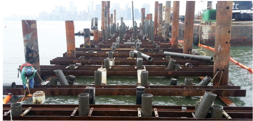
Progress during the project
