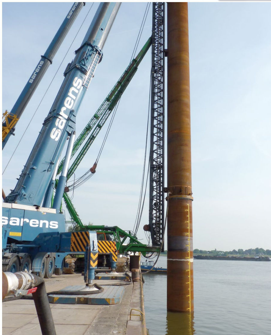
A 2.2-metre BLUE prototype driving a 2.2-metre pile during near-shore tests in August
