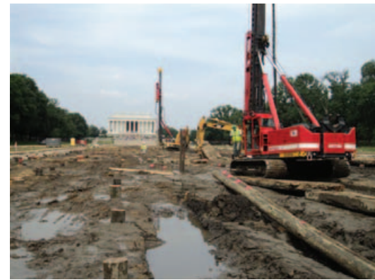
From left: Conditions in 2W, looking W; Crane Mat in 1E with Pile Cut-off Stabilizer; PM-16 driving in 1E.
