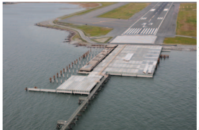
Photos courtesy of JF White Contracting Co.
