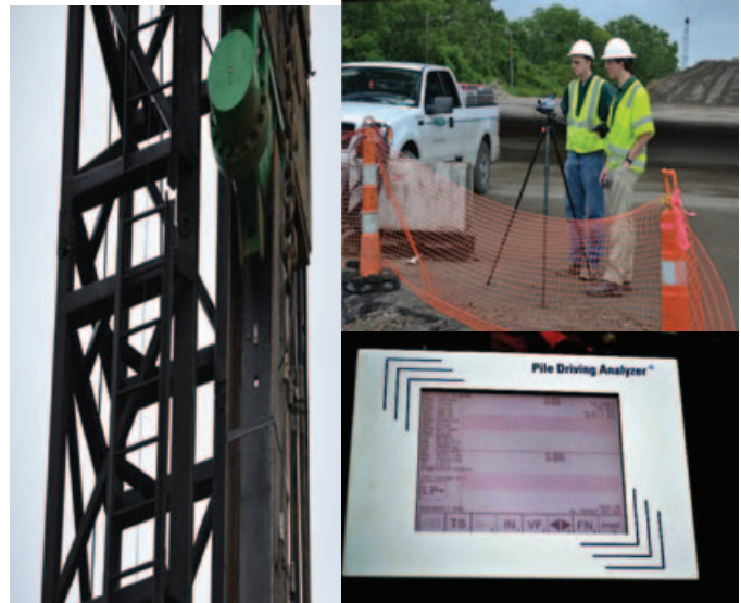
Figure 3: PDA instrumentation on an HP 18x204 and GRL Engineers' Dr. Brent Robinson (left) and Eric Bogen video recording while the PDA Model PAX processes the pile data.
