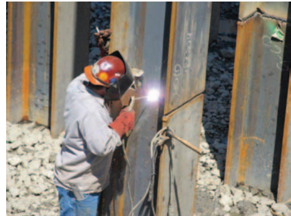
A construction worker welding the piles.
