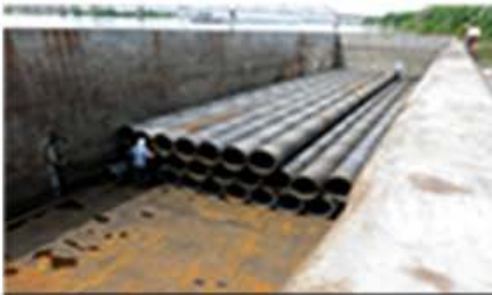
Seabrook Gate Complex (New Orleans, LA)
