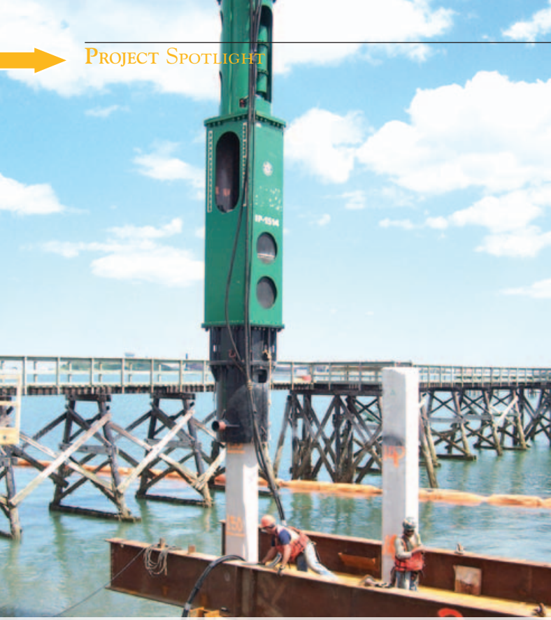
ICE's IP-1514 with off shore bonnet driving 18"sq PCPS piles. These hammers were built new for this job, in Korea, and shipped to JFW on time for the start of the Logan project.
