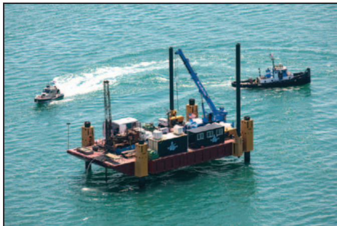
ICE's IP-1514 with off shore bonnet driving 18"sq PCPS piles. These hammers were built new for this job, in Korea, and shipped to JFW on time for the start of the Logan project.
