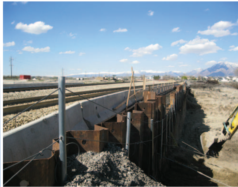
Sheet-pile shoring supporting the Phase One bridge during construction of Phase Two
