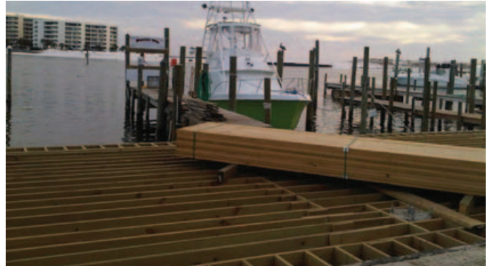
Upgraded treated timber substructure
