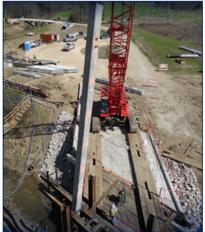
Sheeted jacking pit for the Albany Wastewater Treatment diversion pipe
