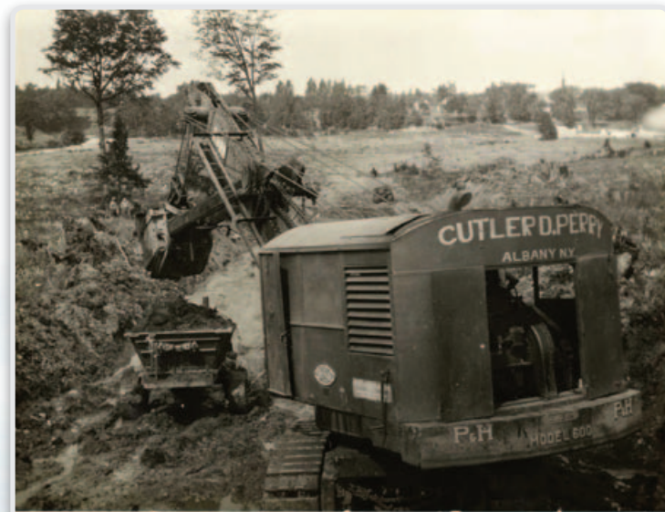
Early days of C.D. Perry, site excavation in upstate New York
