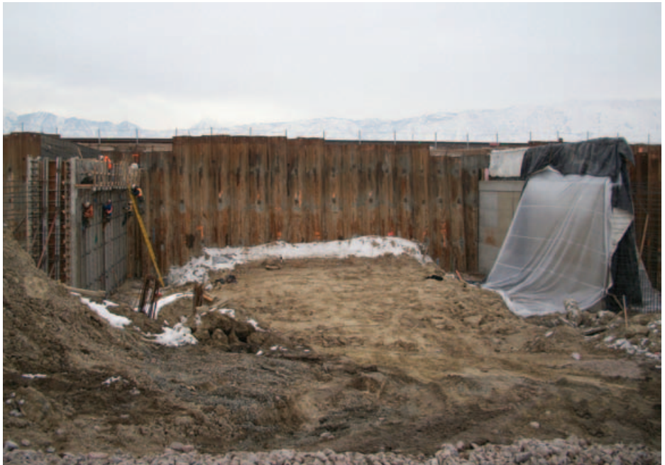
Supporting the existing rail line during Phase One of bridge construction
