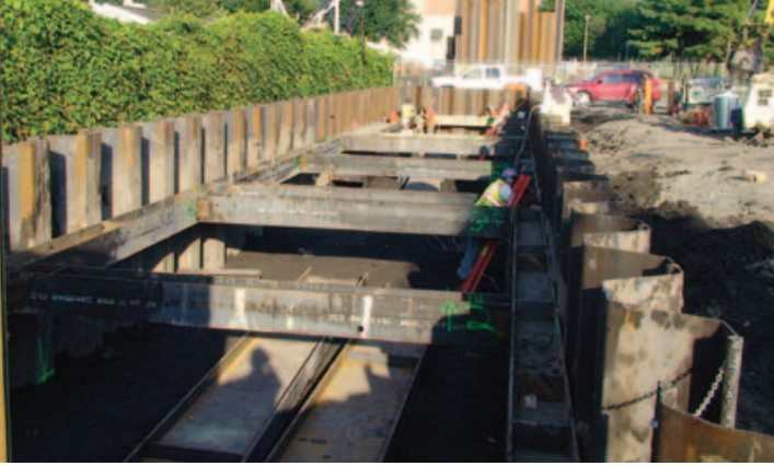
Sheeted jacking pit for the Albany Wastewater Treatment diversion pipe
