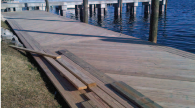
Newly renovated EcoLife stabilized weather-resistant wood walkway
