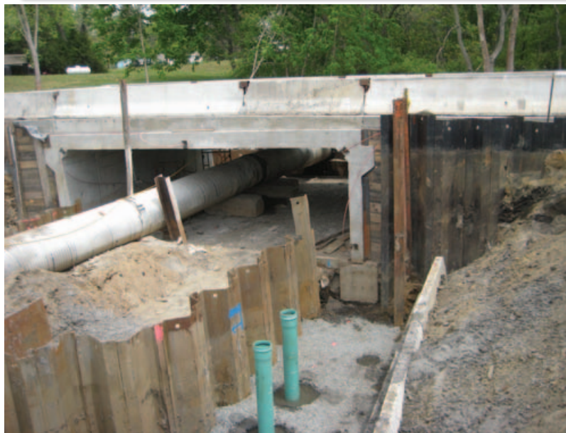
Bridge sheet piling
