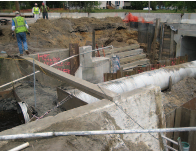
Bridge sheet piling
