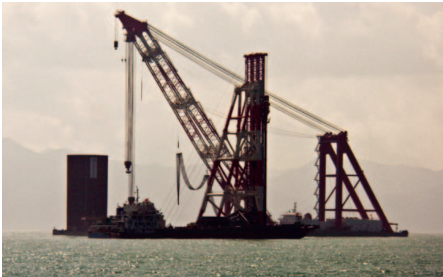
A crane set to pick and drive a 500-ton pile
