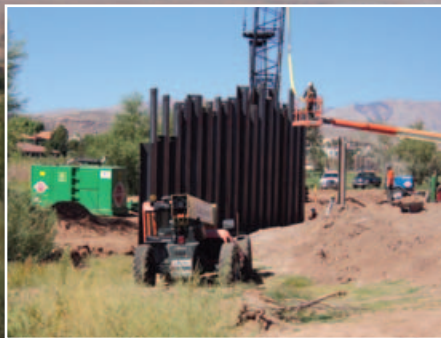
Above: Crews working on installing sheet piling for the project
