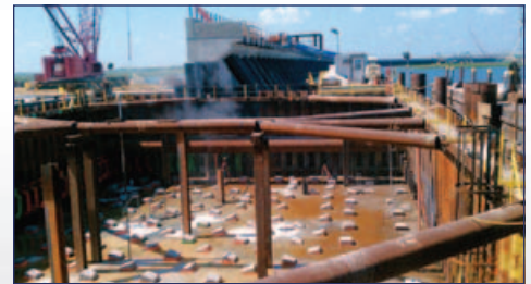
Inner Harbor Navigation Canal Surge Barrier (New Orleans, LA)
