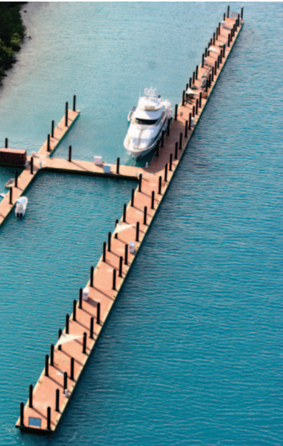
Above: HDPE sleeves were used at Yacht Club Costa Smeralda in the British Virgin Islands
