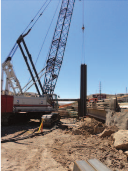
Installing sheet-pile scour protection wall along Santa Clara River
