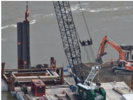
The reconstruction in Fortescue Missouri from the flooding in 2010.
