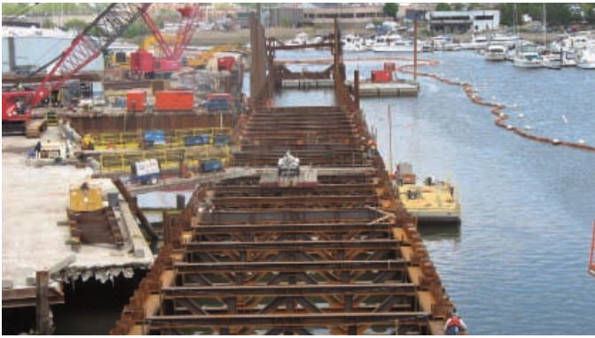
Dura-Bond supplied the fabrication provided the seal welding on sheet and king piles for Mystic River project.
