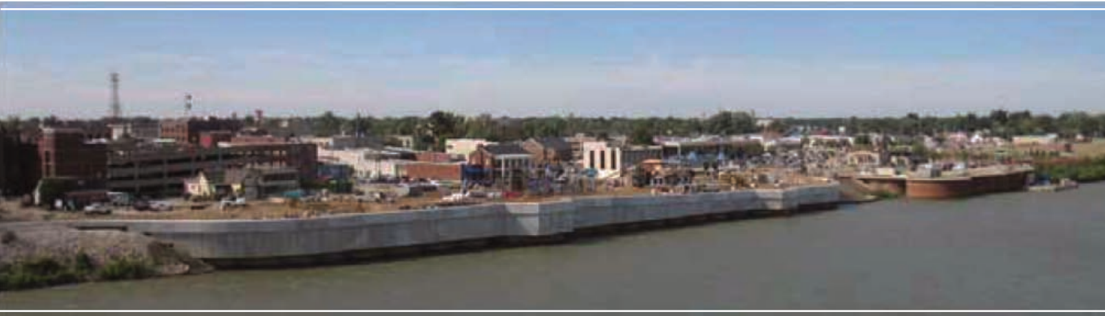
Figure 7. Owensboro Riverwall, Owensboro, Kentucky (2011)
