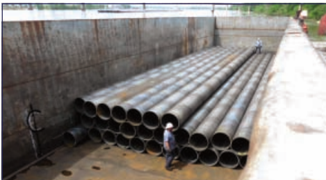
Seabrook Gate Complex (New Orleans, LA)
