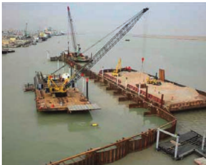
Figure 6. Umm Qasr Seawall, Under Construction (2010)
