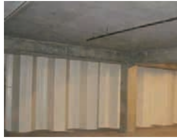
Evo: Los Angeles, CA LEED Silver mixed use development with three levels of below grade parking garage
