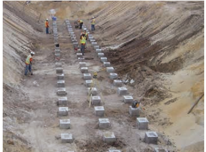
Footing piles for post-tensioned abutment on the John Land Apopka Expressway in Maitland, Florida
