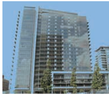
The John Ross Towers: Portland, OR Mixed use development with three level below grade parking garage
