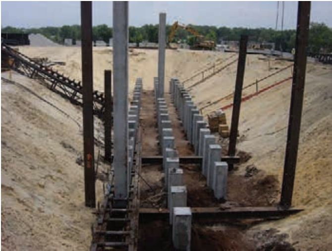
Footing piles for post-tensioned abutment on the John Land Apopka Expressway in Maitland, Florida
