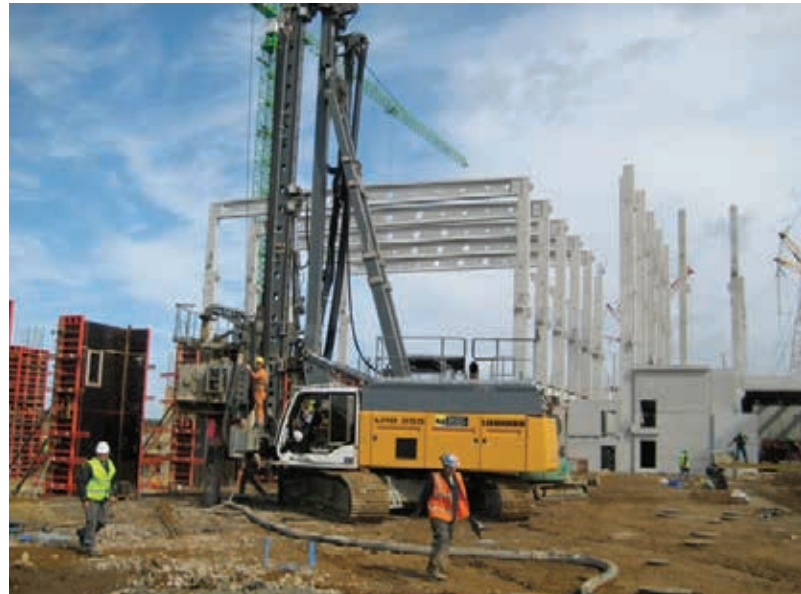
Fig. 4: Liebherr Carrier LRB 255 with Ring Vibrator 32VMR; Photo BVV, Munich
