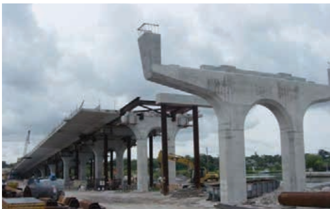
Launching the Deck
