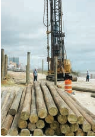
Piling Driven for MB Boardwalk
