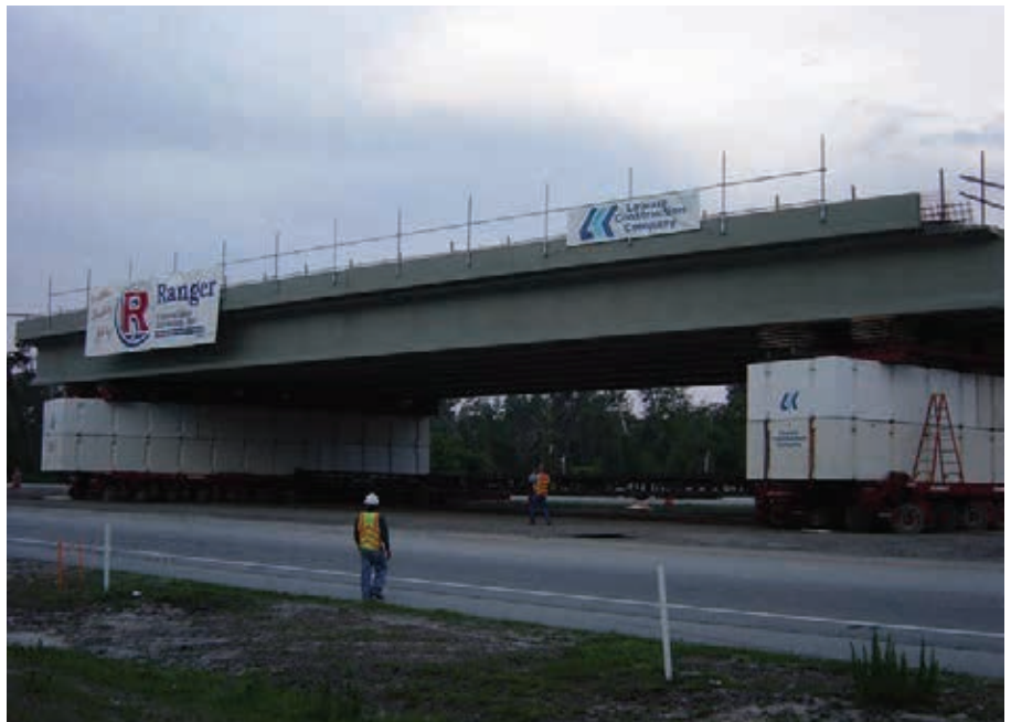
Staging for one of the new spans of superstructure on Graves Avenue over I-4
