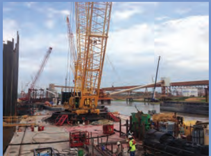
Figure 1 – Ringer crane barge at wharf superstructure
