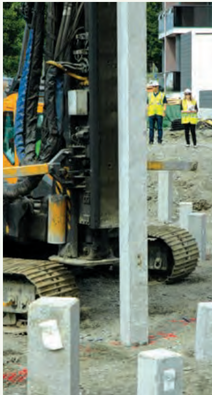
Upper Photo: The Junttan brand is one of the most well known in the pile driving industry. Lower Photo: About 65 percent of all piles driven in Scandinavia are pre-cast, non-prestressed concrete piles.
