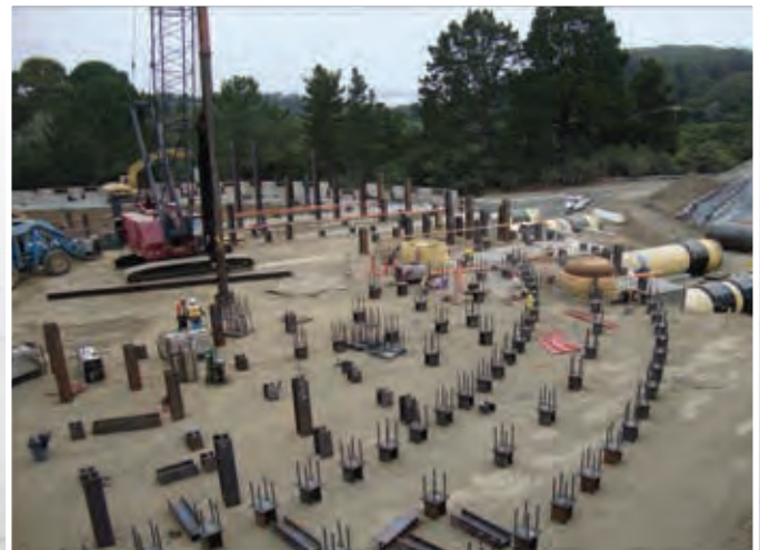
Below: Each pile had to follow the tank wall radius
