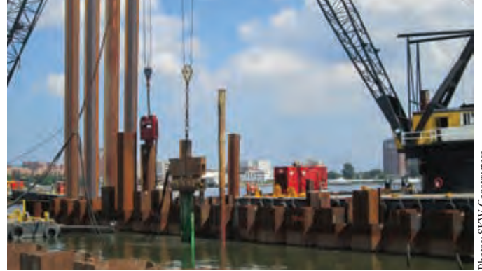
The installation of sheet pile between king piles
