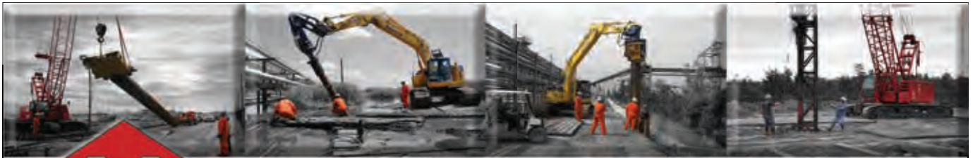
Installation of HP12x53 stabilization pile by CPM Constructors using an H&M 1700 vibratory hammer supported by a Link Belt LS-318 crawler crane
