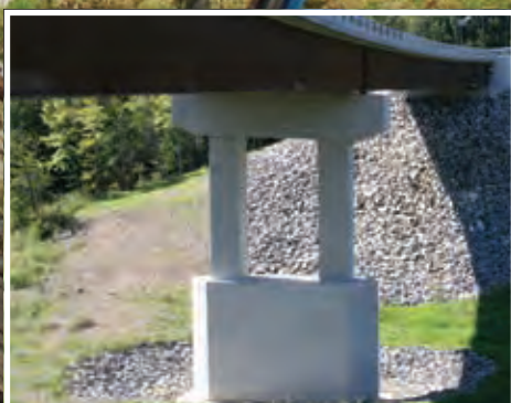
Completed Mile Brook Bridge replacement
