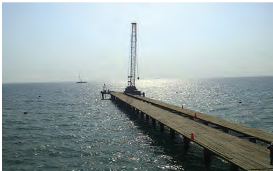
Provisional service pier
