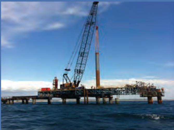
American 9310 in gantry travel positioning pile prior to driving
