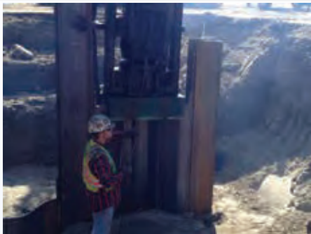
Installing the pile
