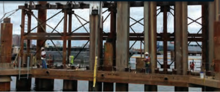
A view of the king pile template
