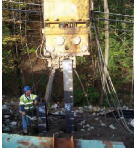
Installation of HP12x53 stabilization pile by CPM Constructors using an H&M 1700 vibratory hammer supported by a Link Belt LS-318 crawler crane
