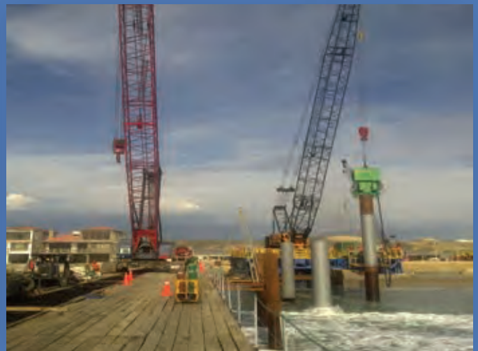
Left: Service pier 110-ton crawler crane.
