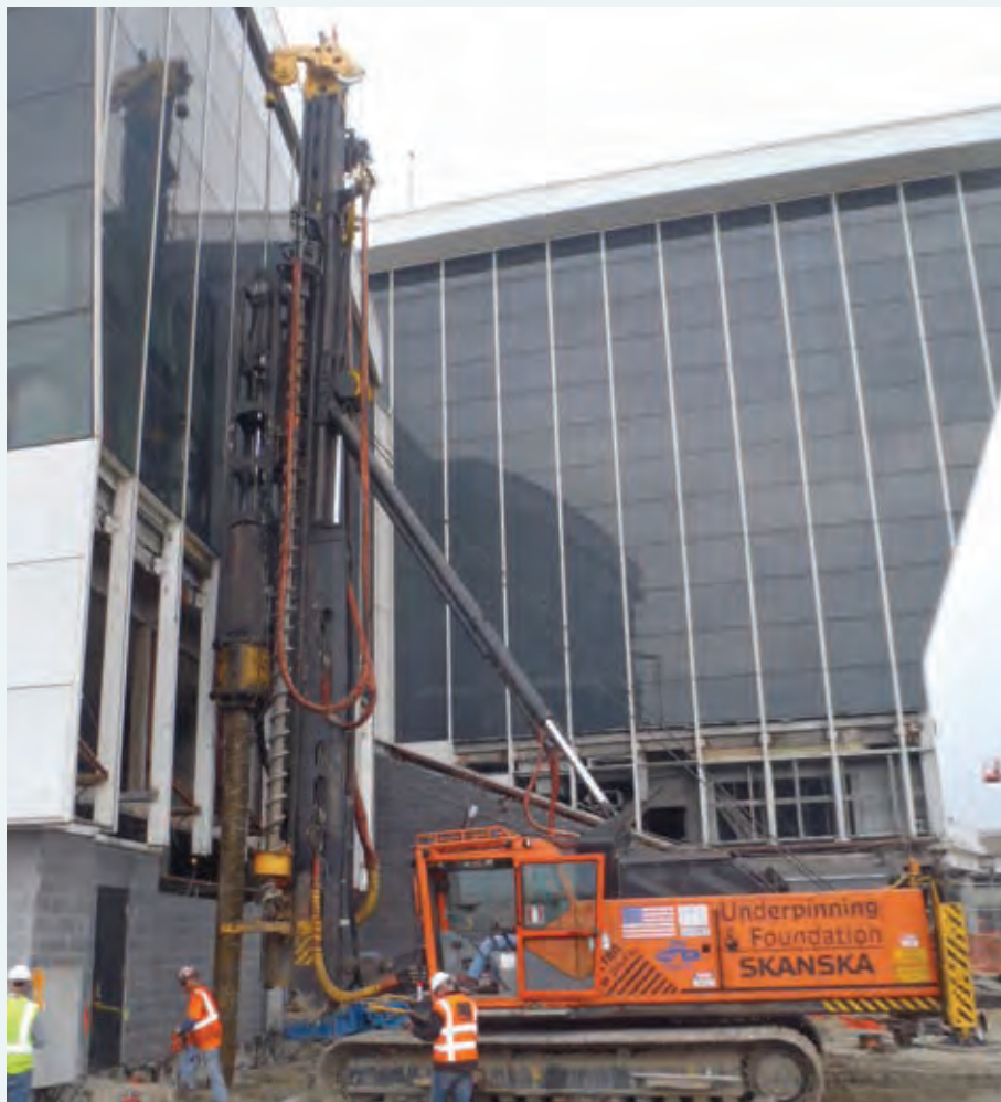
Fig. 3. Driving a battered pile next to the terminal
