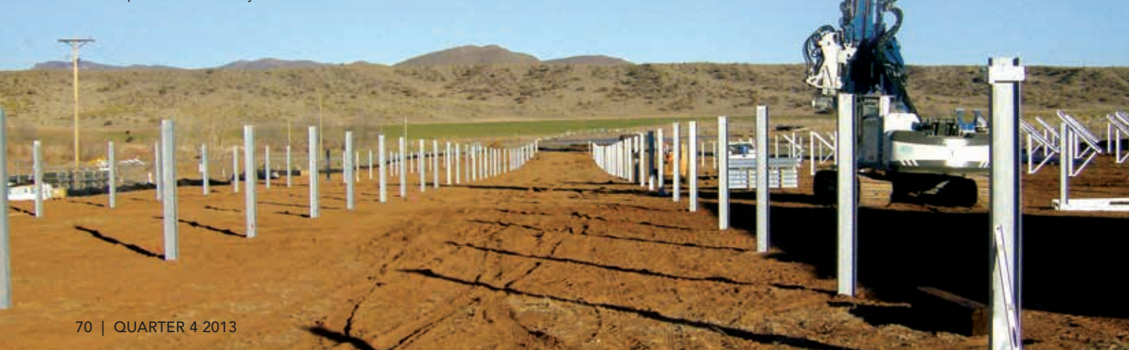
Steel posts for solar arrays
