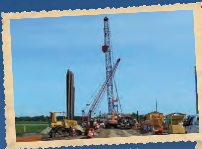
Cape Romain Contractors are currently working on a multi-bridge replacement project
