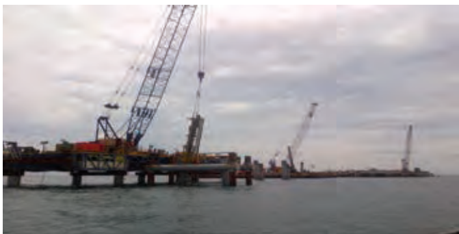
Driving battered piles
