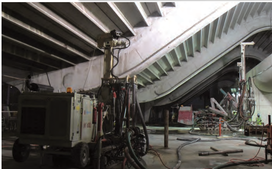
Work progresses on the Port of Miami Tunnel project
