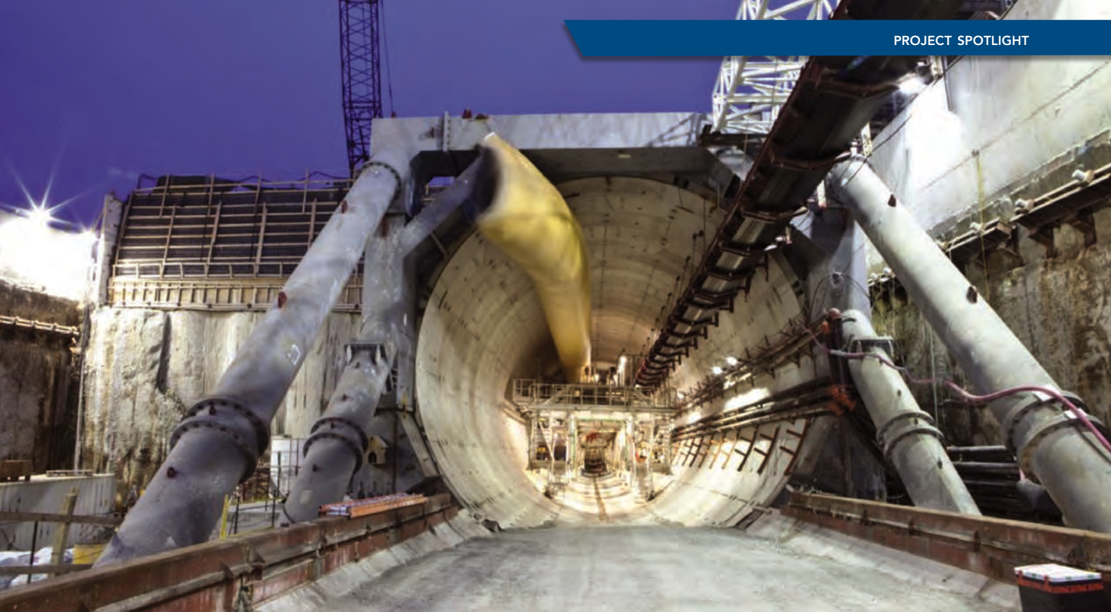
A view of the tunnel entry
