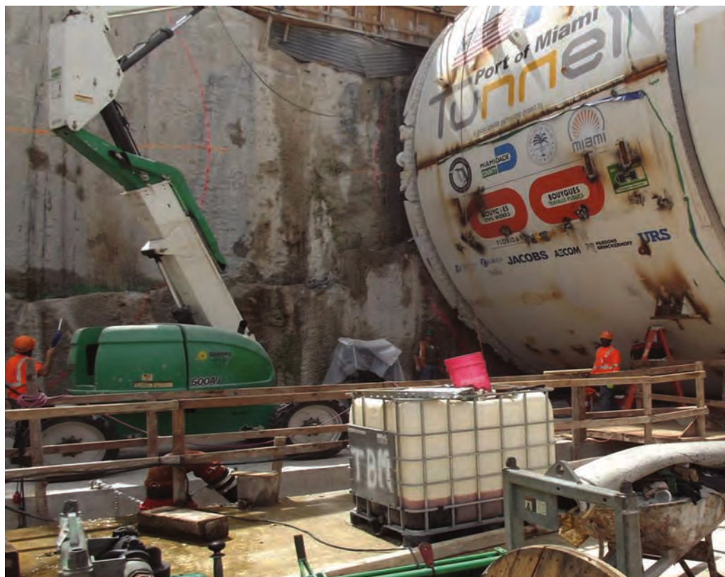
Working on the Port of Miami Tunnel project
