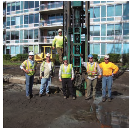
Working to drive piles for the Hudson River Walkway
