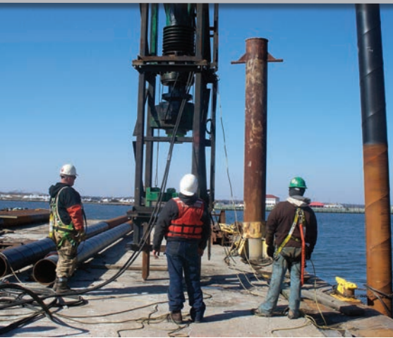
Workers on the jobsite at Cape May
