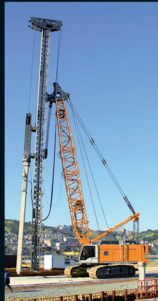
The Liebherr LRB 255 on site and in operation in Quebec, Canada
