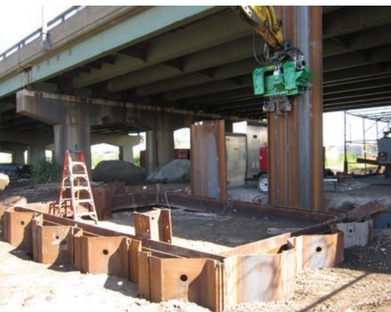
Figure 1: Sheet pile driving with ICE® 6e in low overhead situation
