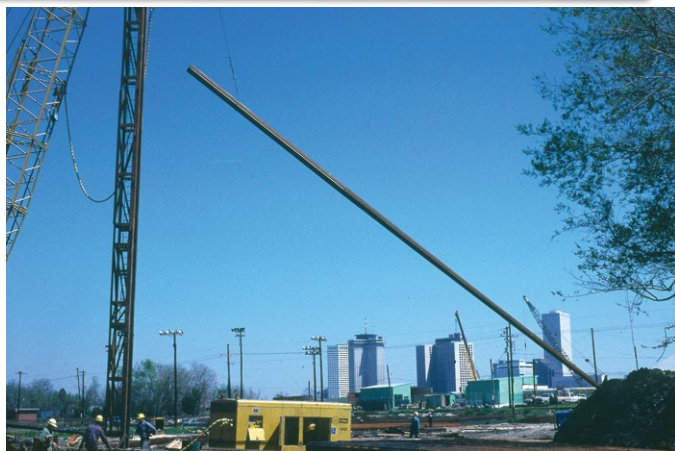
7.625-inch x 16-inch x 100-foot-long Monotube pile
