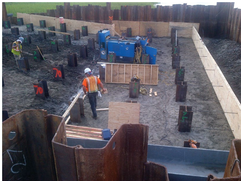
Driving piles and then installing a heavy reinforced concrete slab atop those piles addressed job site challenges in a positive way
