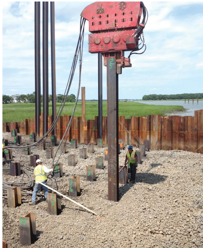
Vibration of a steel H-pile
