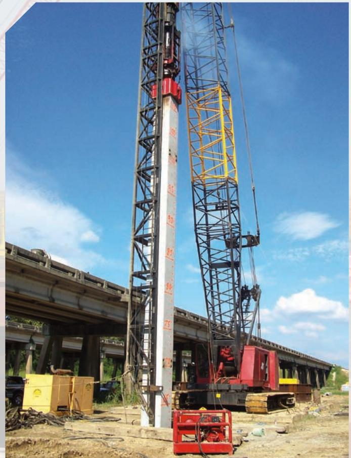
Logging square, precast concrete pile at I-12 Widening
