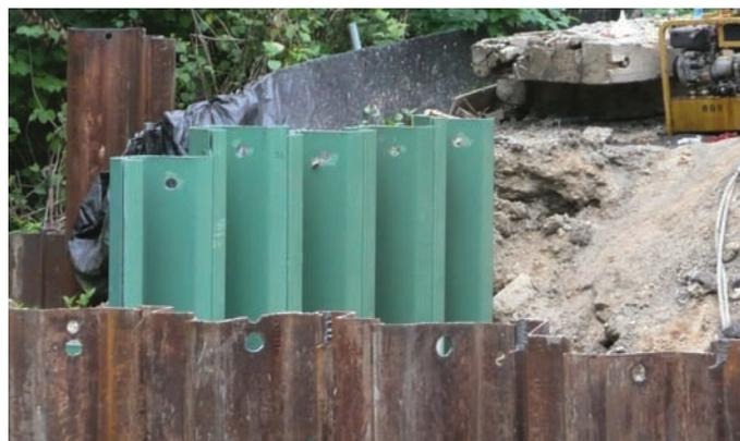
Sheet piling just after installation at the Tuckahoe Creek Bridge between Easton and Denton, Md.
