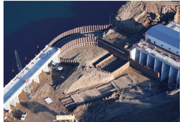
the 30-foot deep excavation. Construction progress was challenged by the unusually wet November and December of 2010 and exceptionally hard Tehama formation, where the standard penetration resistance was as high as 50 blows per .3 of a foot.
