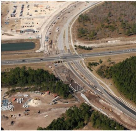
The construction of two-thirds of a mile of road and two bridges at Plantation Oaks Boulevard, using, among other things, 1,700 linear feet of prestressed concrete pile
