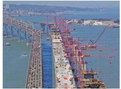
an earthquake. Support for the tower includes a massive marine foundation consisting of 13 drilled shafts extending 196 feet below the water surface anchoring into the bedrock. Support for the eastern end of the SAS includes another massive marine foundation that extends 340 feet below the surface. Supporting the western end of the SAS is a land-based foundation that is drilled down 80 feet into Yerba Buena Island.
