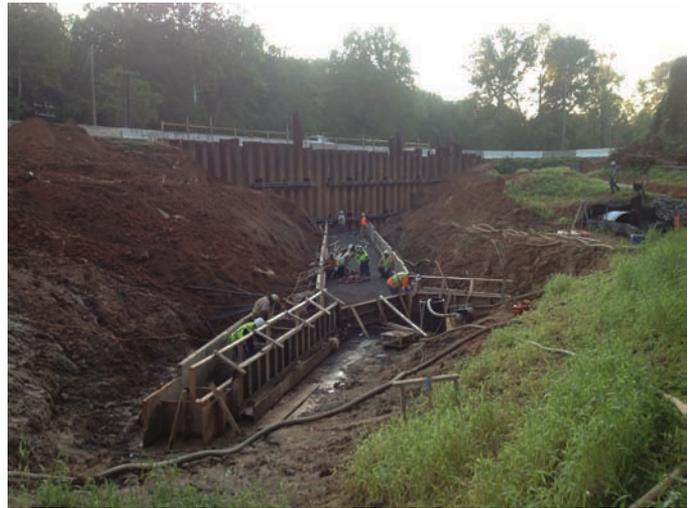
Temporary PZ-27 sheet piling for NC DOT on Highway 220 in Guilford County, N.C.
