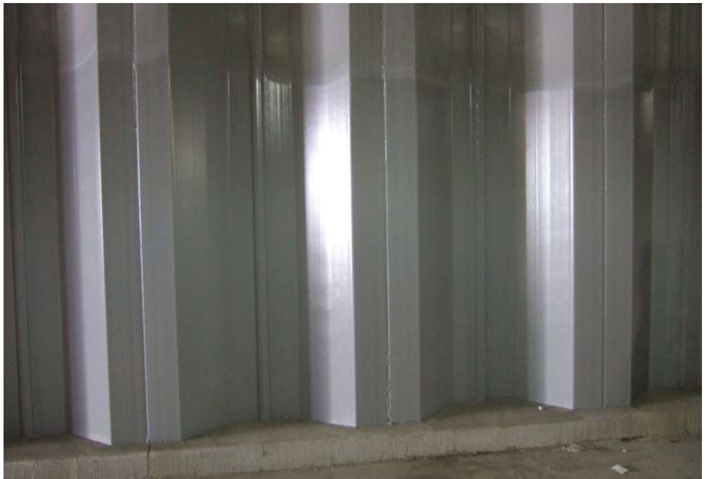
Floor / wall interface connection
