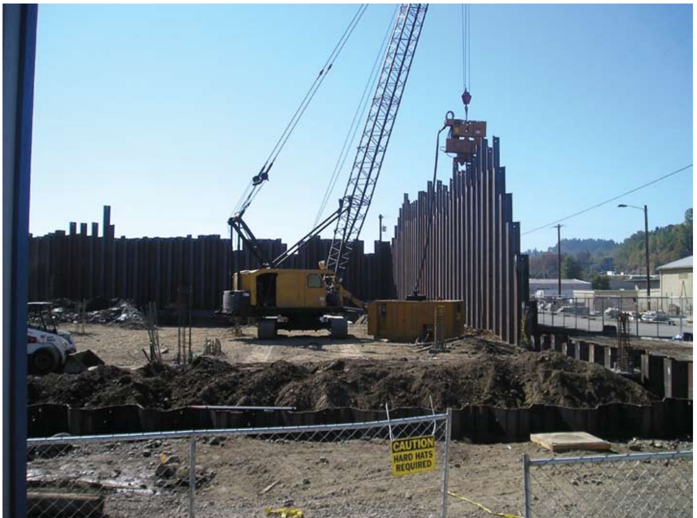
Conventional hammer installation for permanent sheet pile wall
