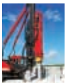
On the Cover: Junttan rig driving concrete piles
