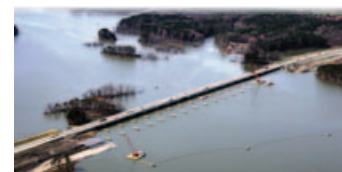
On the Cover: Aerial East Bound and Existing Pier Caps for the 1-80 Widening over the Meander Reservoir by The Great Lakes Construction Co. (submitted by Jeremy Levenson and Randy Radel, GLC)
