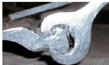
Steel sheet pile locks filled or being filled with sealant
