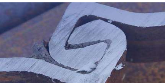
Steel sheet pile locks filled or being filled with sealant
