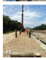
A Manitowoc 999 using an elevated template and the ICE IP-1514 to drive a 180 foot long precast pile on the Boston-Logan International Airport Runway 33L.
